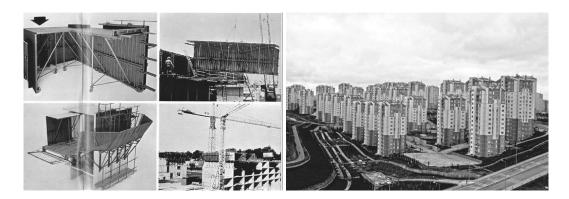
Figure 3.34. (left) The use of formwork half-tunnel construction system<sup>250</sup>
