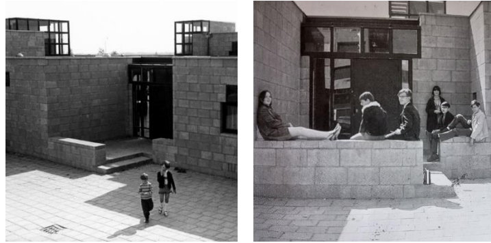
Figure 3.30. The entrance as the in-between realm in Montessori School (Accessed December 24, 2021 from https://www.ahh.nl/index.php/en/projects2/9-onderwijs/114-montessori-school-delft ; Hertzberger 1991/2001, 33)
