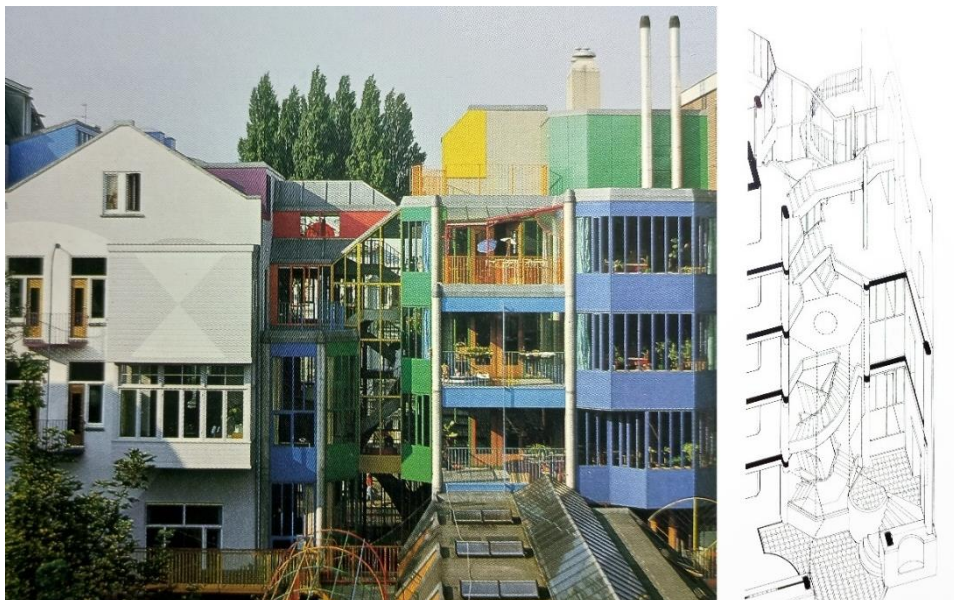
Figure 3.13. The spiral staircase between old and new building of Hubertus House, Home for Single Parents and their Children [1973-81] (van Eyck 1999, 193-194).
