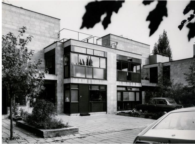
Figure 3.27. Diagoon Dwellings (Accessed December 26, 2021 from https://www.ahh.nl/index.php/en/projects2/14-woningbouw/79-diagoon-experimental-housing/ )
