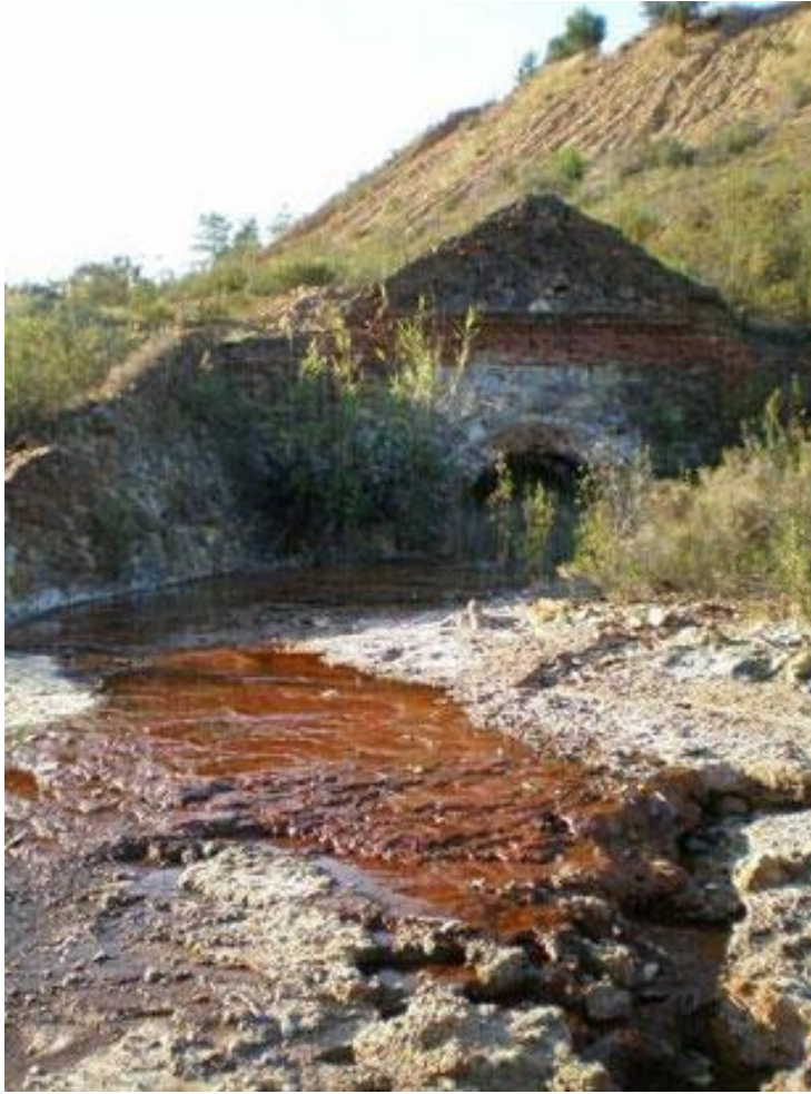
Figure 2.6. AMD formation at Roman-era portal in Spain (INAP, 2014).
