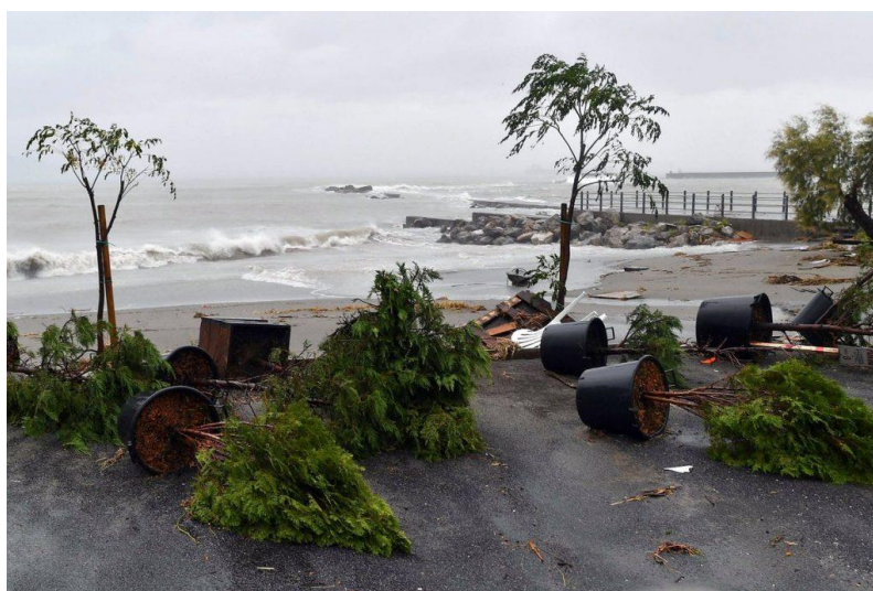
Figure 7.9. Damage from Medicane Zorbas in Greece, September 2018
