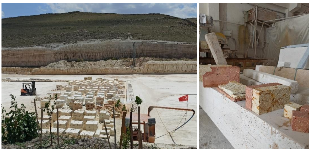
Figure 3.2. General view of the stone quarry near Karadağ Region in Avanos (Nevşehir, Turkey) (left), the tuff types cut to size in the stone cutting unit of the quarry (right).
