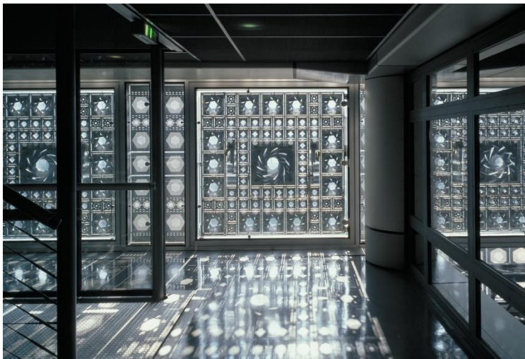
Figure 2.8. The facade system, like the camera lenses of Institut du Monde Arabe (Schielke, 2014)
