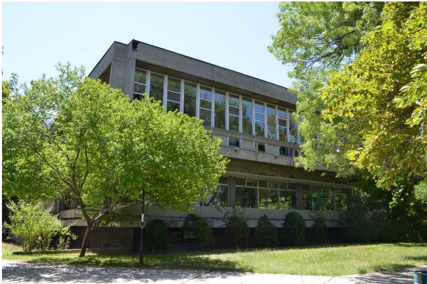
Figure A.4 Exterior view of the north section of the METU Cafeteria Building, pictured by the author
