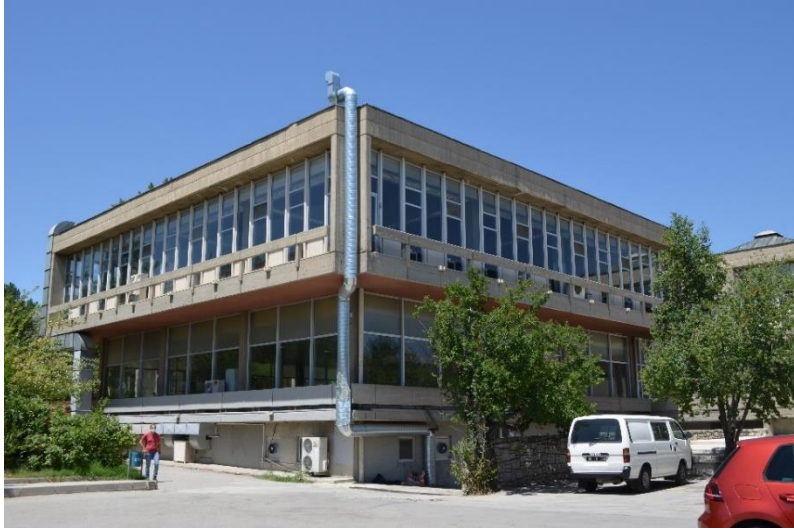
Figure A.1 Exterior view of the south section of the METU Cafeteria Building, pictured by the author
