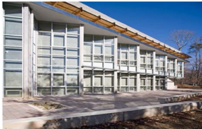
Figure 2.6 Zigzag Trombe Wall , Residential structure built near Asheville, North Carolina (Sokol, 2008)
