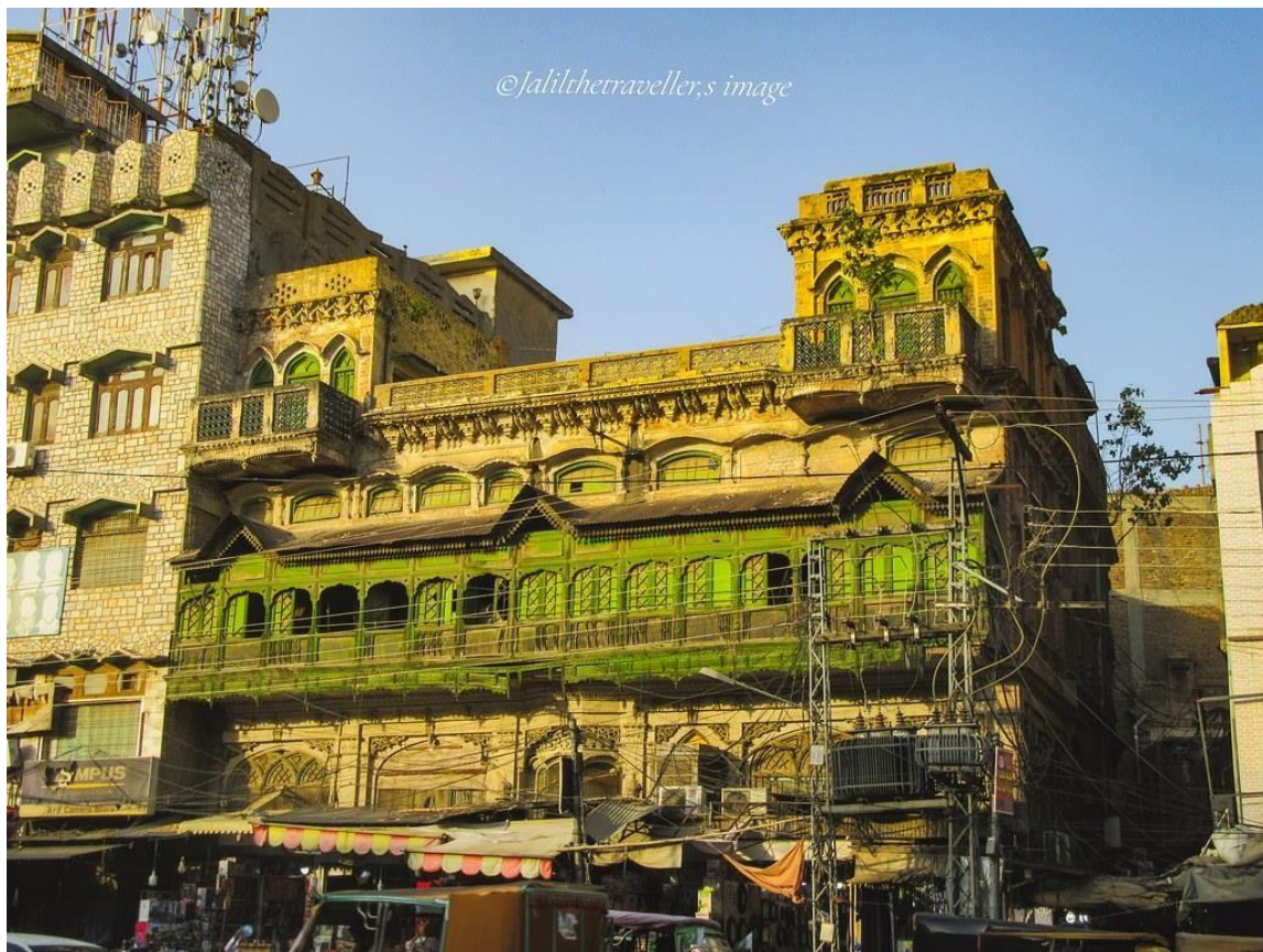
Figure 8: Colonial British Mansion in Raja Bazaar Rawalpindi (Courtesy: Jalith Travellers)
