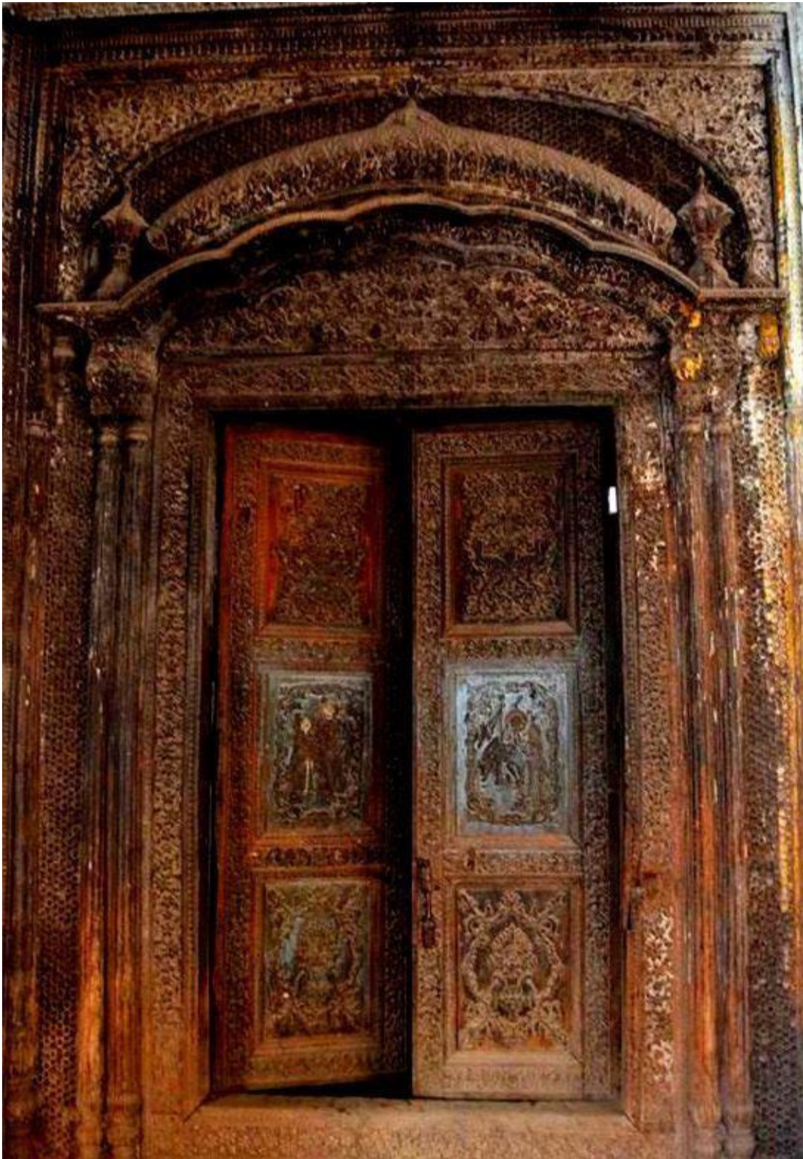
Figure 43: Haveli's main entrance door from the street. (Courtesy: The Main Door (By S. Hassan). (2012). Shiraz Hassan Blogspot. http://shirazhassan.blogspot.com/2012/07/haveli-soojan-singh-crumbling-heritage.html )
