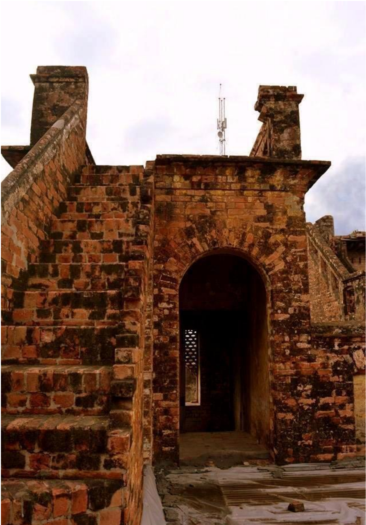
Figure 49: Staircase to terrace from room 314c. (Courtesy: (By F. Khan), (2018). Feroza Khan 23 Blogspot. http://ferozakhan23.blogspot.com/2018/05/ )
