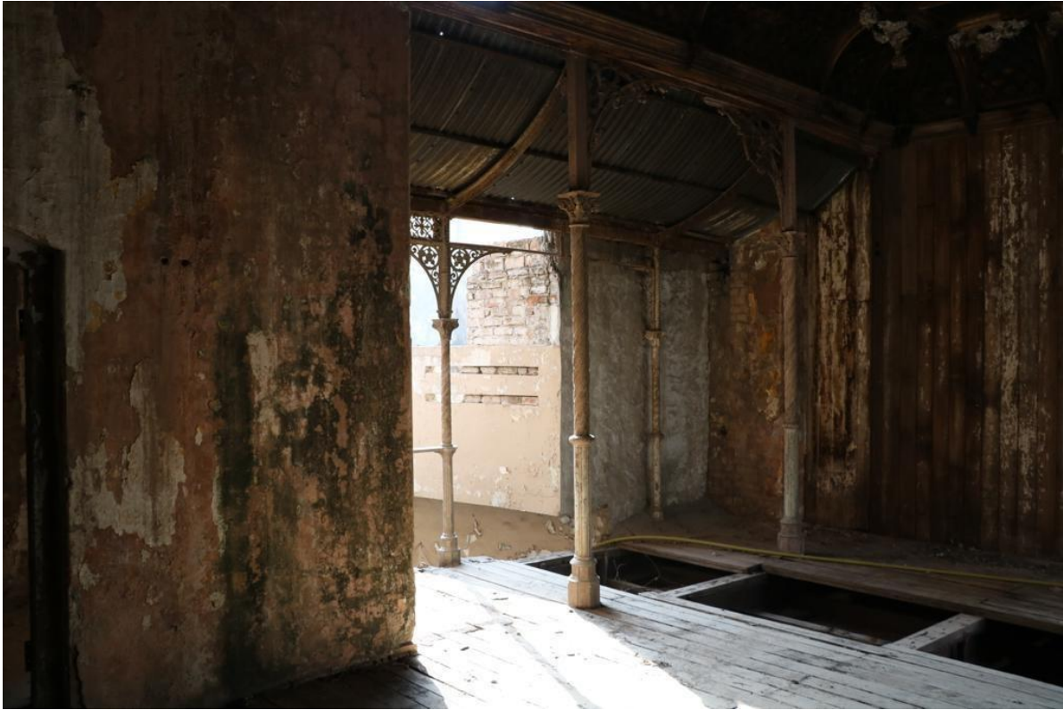
Figure 53: Bridge deck showing pitched roof. (Courtesy: Rogers Kolachi Khan & Associates (Ltd.), Assessment of the Existing Condition at the Historic Haveli Sujan Singh, Rawalpindi, Pakistan )
