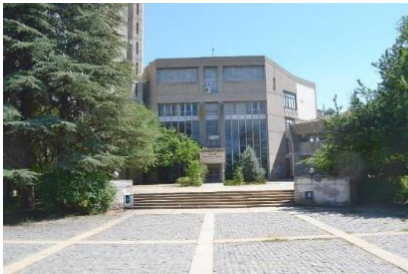
Figure 53. Photograph focusing on Central Engineering Building by the author
