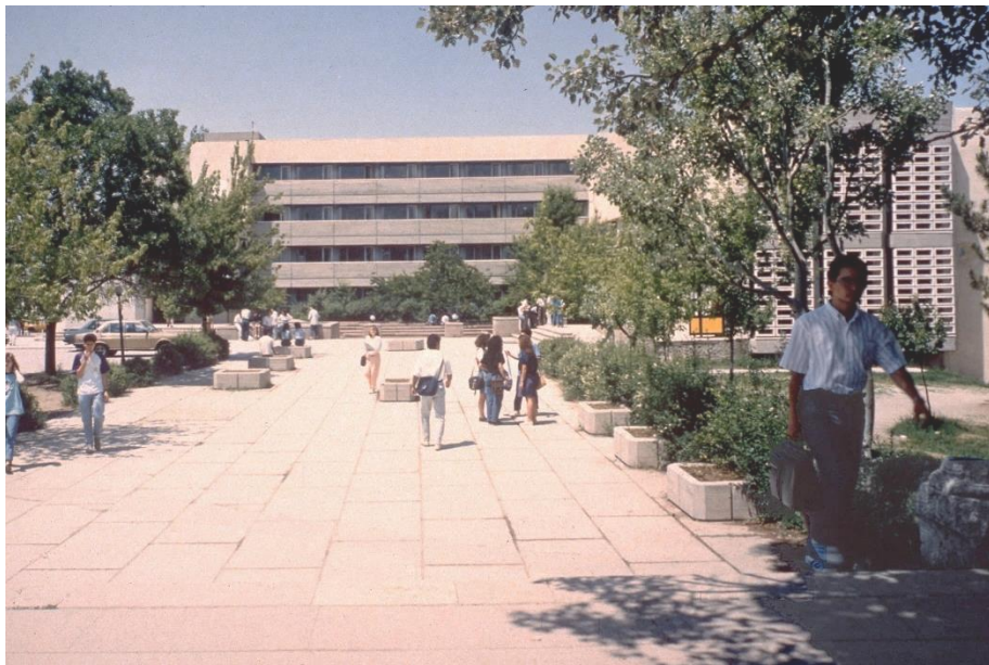
Figure 96. Photograph of Administrative Sciences Faculty Building, source: salt archives
