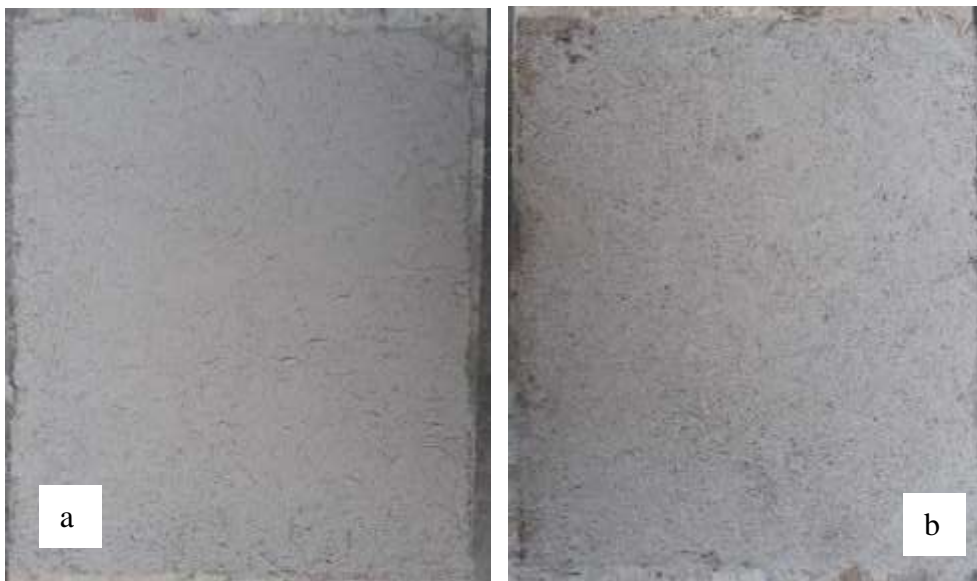
Figure 6-16: Specimens of mortar Ka000207-221001 (a) and Ka000210-221001 (b) with the surface cracks visible on mortar Ka000207-221001.
