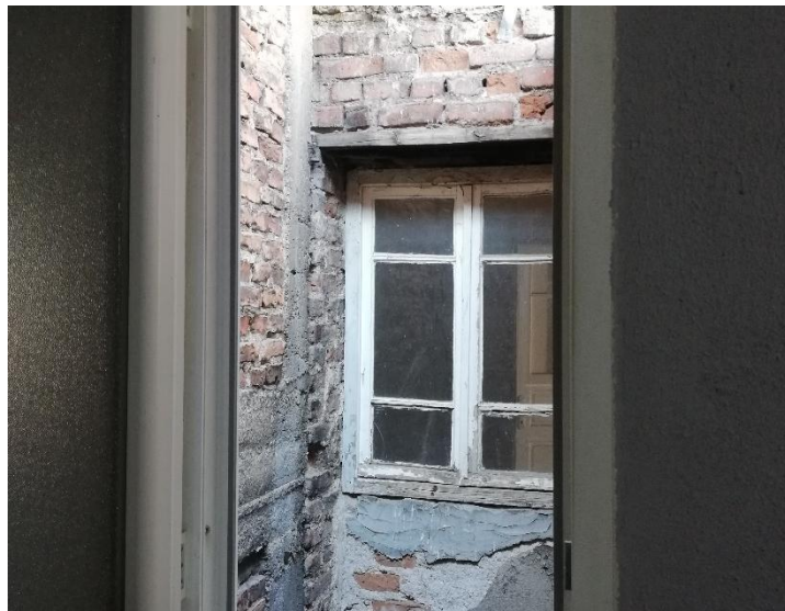
Figure 3.12. Building B, window facing ventilation shaft. (Author, 2022)
