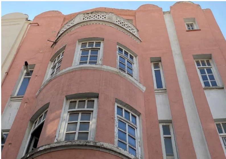
Figure 3.26. Mevsim Street façade of Building A (Author, 2021)
