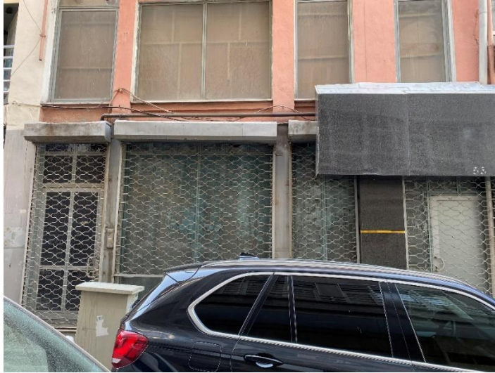
Figure 3.25. Mevsim Street façade of Building A (Author, 2021)
