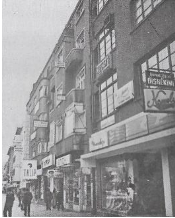
Figure 3.3. Photograph of Foto Apartment, Seyfi Arkan, 1935 (Aslanoğlu, 2001)
