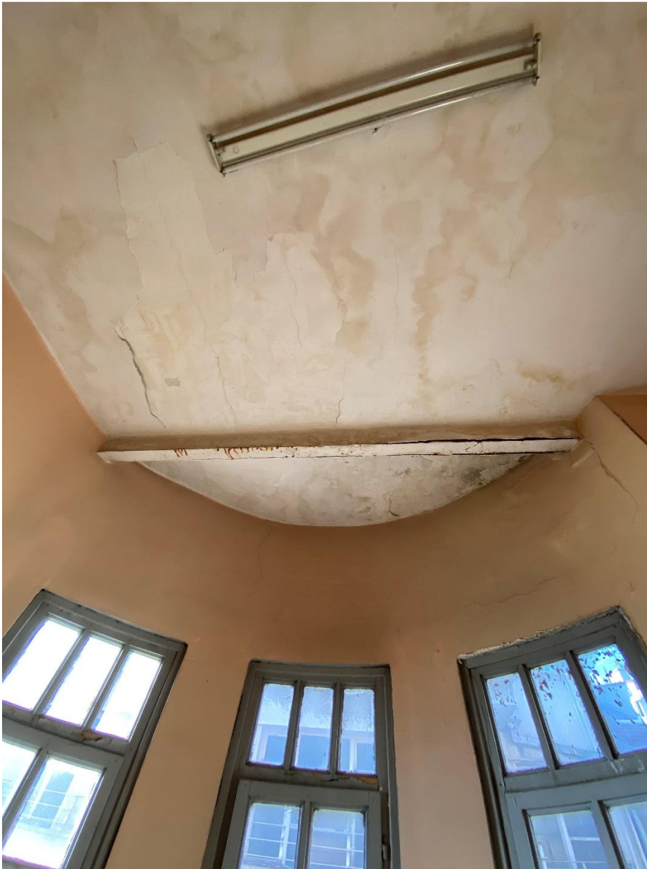
Figure 3.28. Third floor steel beam of Building A (Author, 2021)
