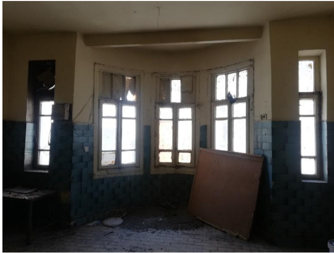
Figure 3.37. The windows on projection in first floor of Building B (Author, 2022)
