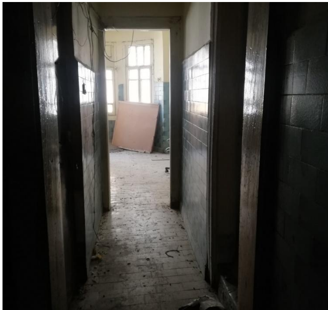
Figure 3.36. Hall on the first floor of Building B (Author, 2022)
