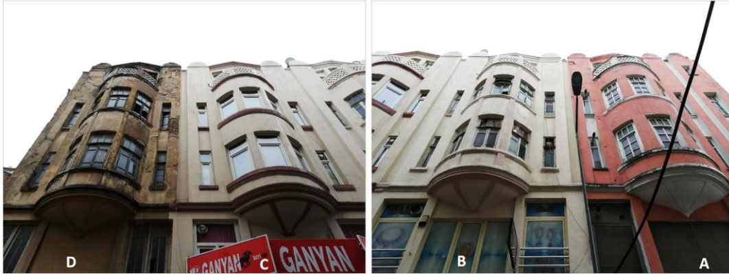
Figure 3.18. Buildings on Mevsim Street, from Konya Street to Anafartalar Street, respectively (Author, 2021)
