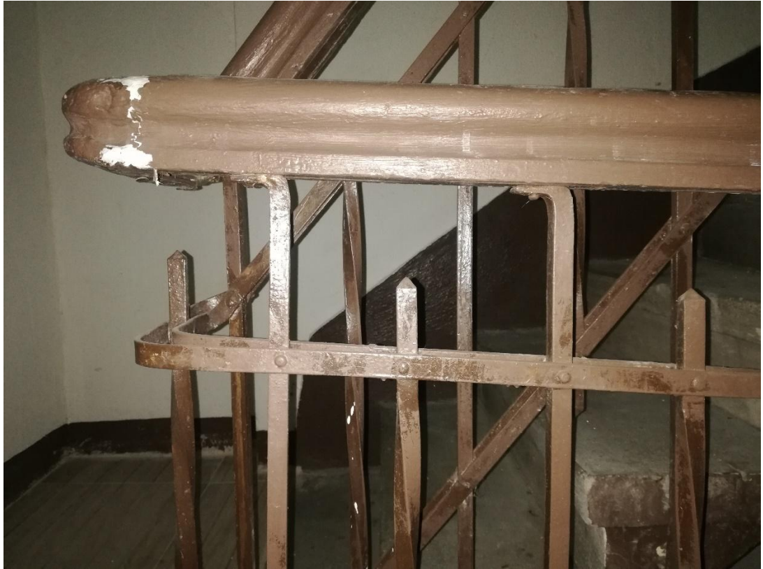
Figure 3.15. Stair railings of Building C. (Author, 2022)
