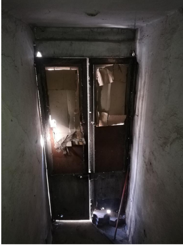
Figure 3.50. Apartment door from inside, Building D (Author, 2022)
