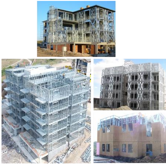
Figure 1.1 CFS structural framing systems
