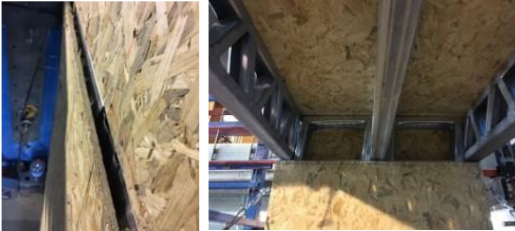
Figure 8.11 Deformations observed at platform framing of specimen WA-5
