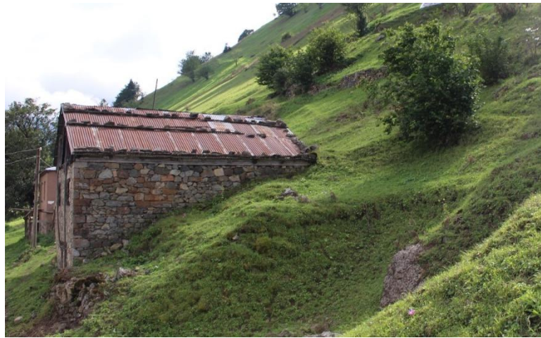
Figure 3.65: Terzili neighborhood, a traditional house set into the slope
