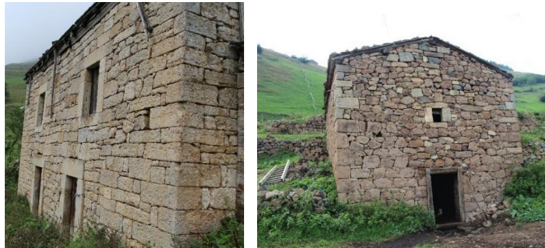
Figure 3.77: Piştöflu neighborhood, doors framed with cut stone (left); Binatlı neighborhood, doors framed with timber (right)
