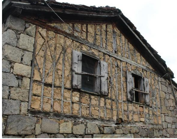
Figure 3.71: Zurnacılı neighborhood, mixture of göz dolma and muskalı technique
