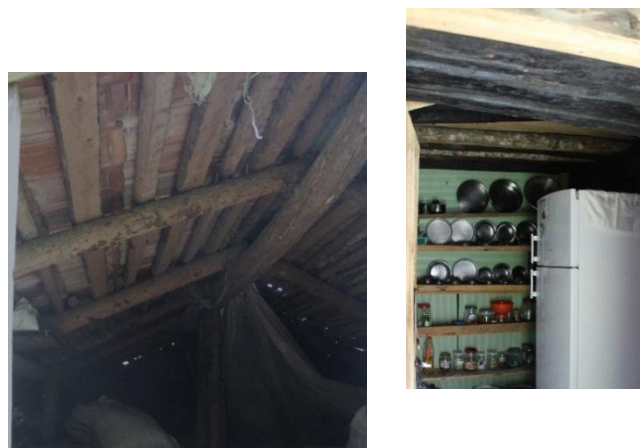
Figure 3.74: Zurnacılı neighborhood, barn, open roof construction (left); Zurnacılı neighborhood, surviving ceiling planks (right)
