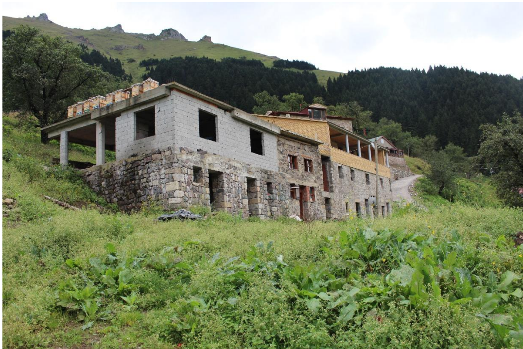
Figure 3.12: Zurnacılı neighborhood, the guesthouse under construction
