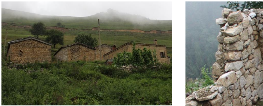
Figure 3.70: Piştöflu neighborhood, stone masonry houses (left); Piştöflu neighborhood, section of a wall of a house
