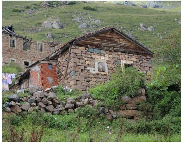
Figure 3.72: İşhanlı neighborhood, horizontal timber panels
