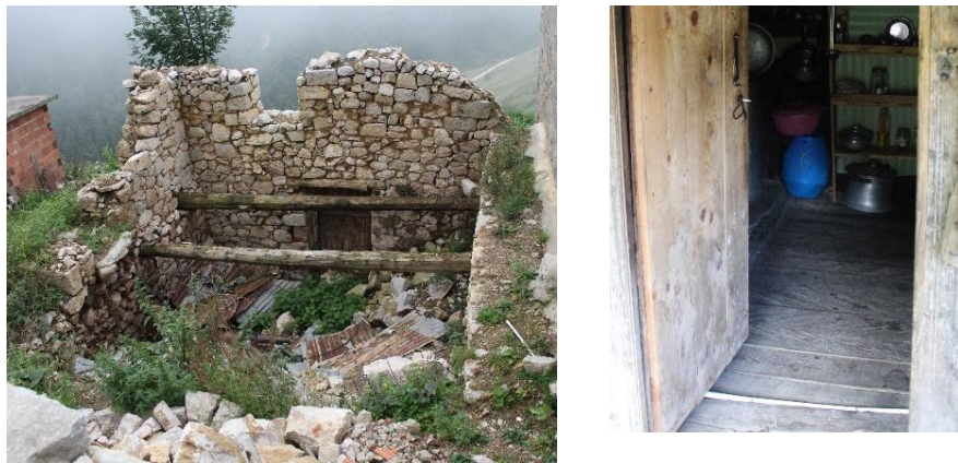
Figure 3.73: Piştoflu neighborhood, timber beams (left); Zurnacılı neighborhood, timber planks (right)
