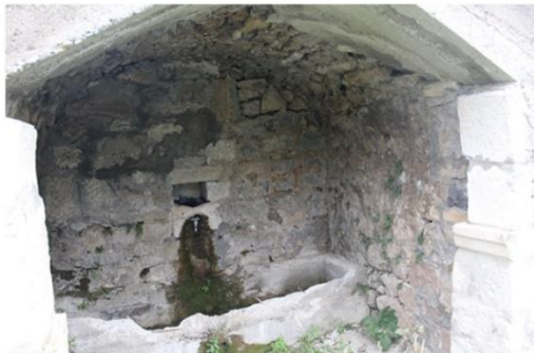
Repairs on F - 3 Fountain
