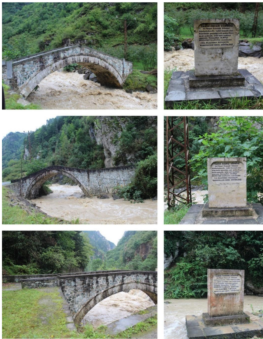
Figure 3.10: Yanbolu valley, stone bridges
