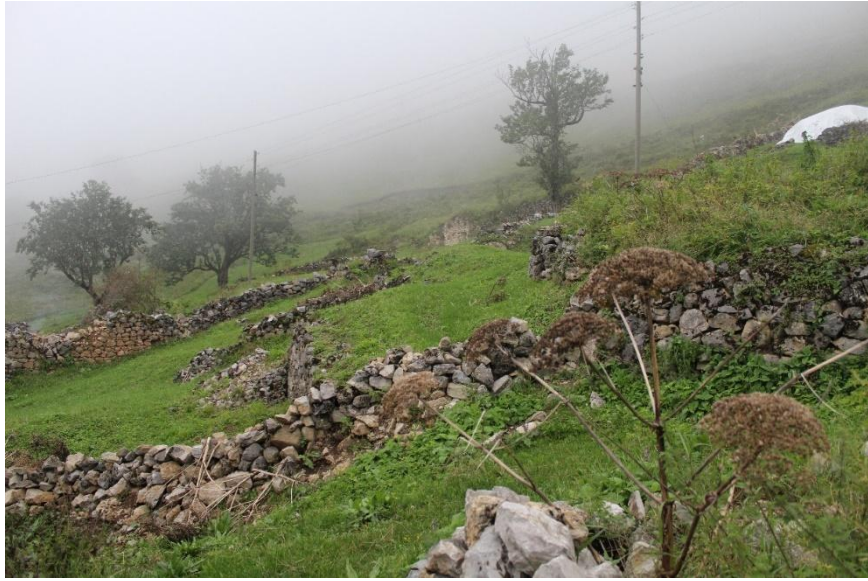
Figure 3.26: Piştoflu neighborhood, the surviving courtyard walls
