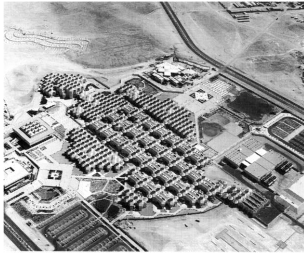
Figure 2.4. The Aerial view of Qatar University by Kamal El Kafeawi, Doha, Qatar completed in 1985 retrieved from the document for Aga Khan Award for Architecture in archnet.org.
