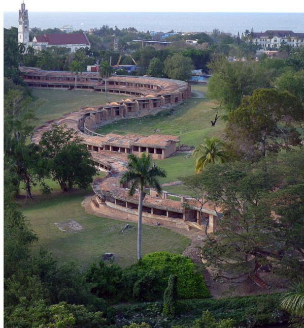
Figure 4.52. View of the School of Music from the CMP Report 2020 p.153
