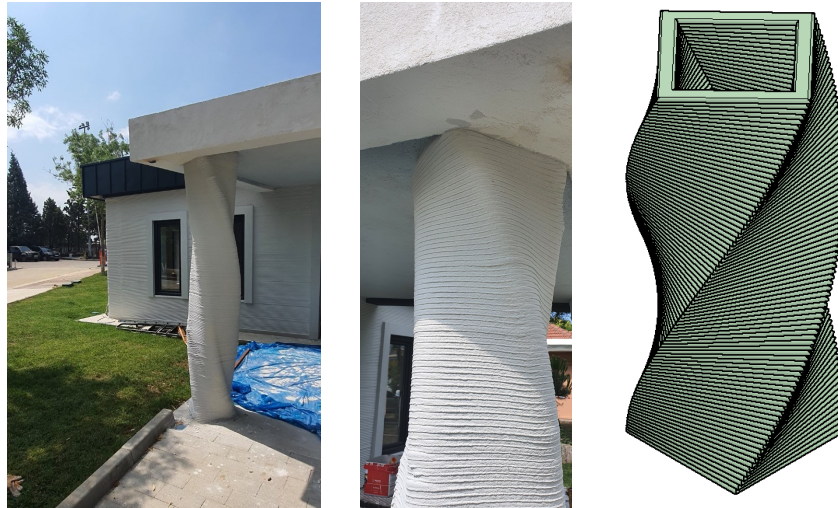
Figure 3.31: An illustration of the column that was printed by İSTON Inc. and its simulated geometry to be utilized in buildability analyses.
