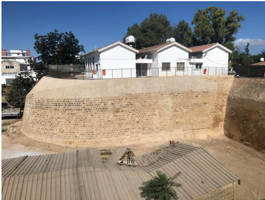
Figure 3.47b. Quirini Bastion after the restoration of collapsed parts. (E. Reis archive 2021)
