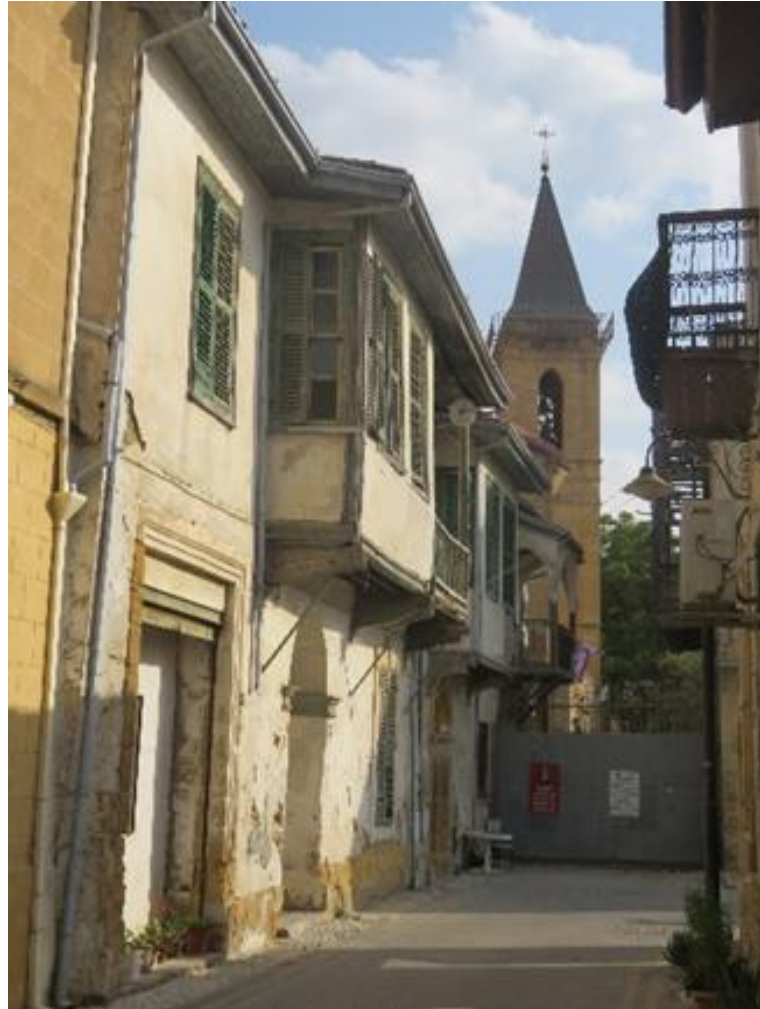
Figure 2.11. Buffer zone from the Arabahmet Area of the northern part of Nicosia (E. Reis archive, 21 August 2016)
