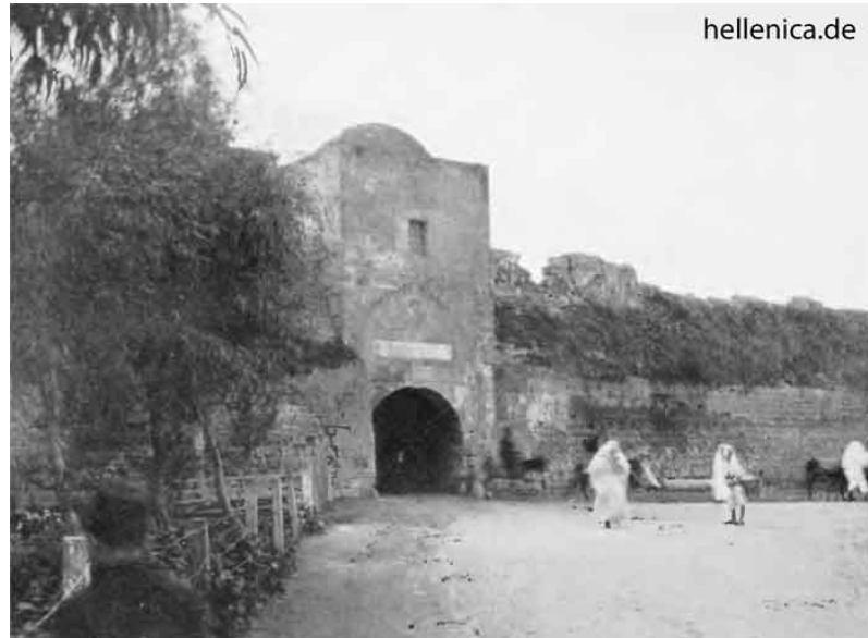
Figure 3.7. Kyrenia Gate before each side cut ( http: www.hellenicaworld.com accessed 20 June 2019)
