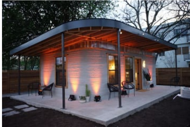
Figure 2.11. The first 3D concrete printed community of houses for low budget construction (Verge, 2018)
