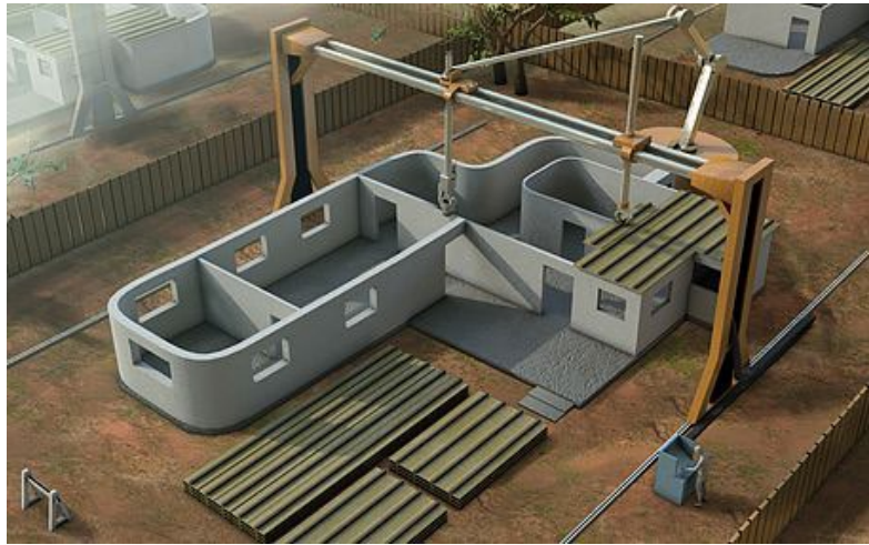
Figure 2.3. Contour Crafting Method (Khoshnevis, 2010)
