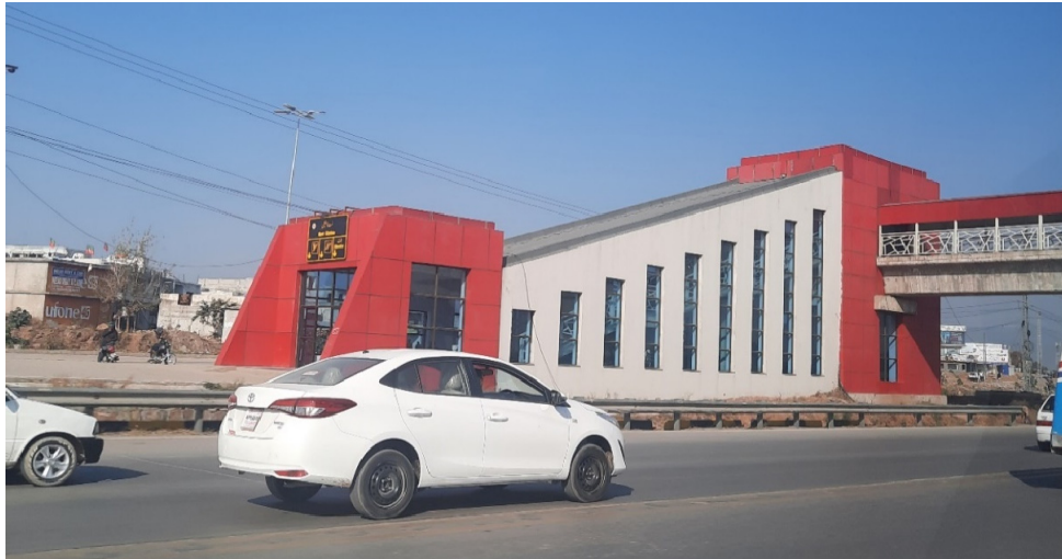
Figure 4.40. Fencing and lack of pavement around BRT station area. Source: Author
