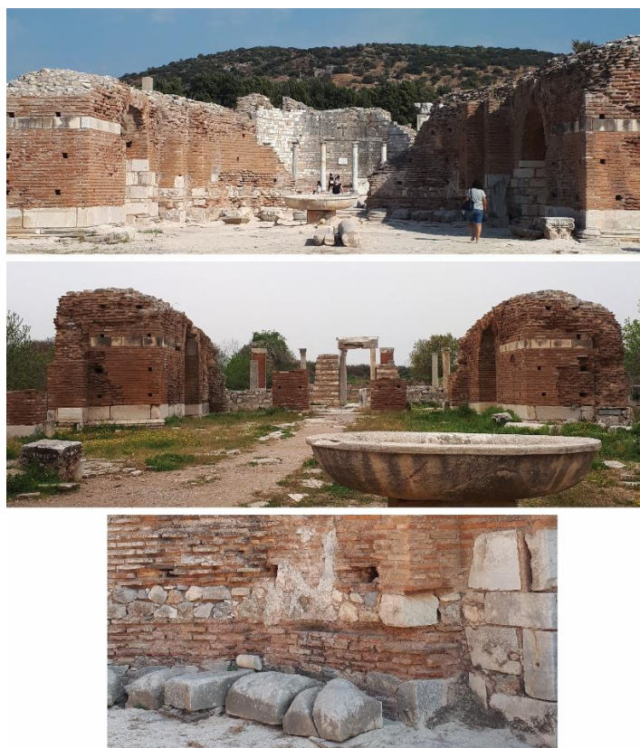
Figure 3.33. The Church of the Virgin Mary, the domed church, nave and aisles (above and middle) and the recessed-brick construction technique (below)
