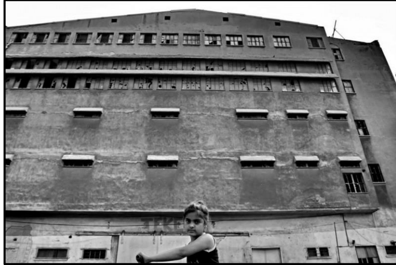
Figure 5.5 Demolished TEKEL Storage Next to Ege Neighbourhood 384
