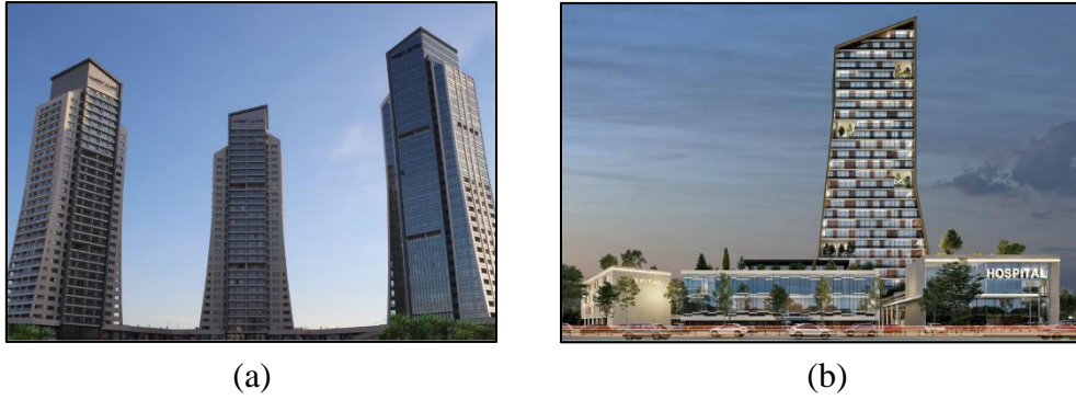
Figure 4.31. (a) West Gate Residence Blocks, (b) Incek Health and Living Center Sources: http://www.msamimarlik.com.tr/projeler/karma-kullanim/west-gate_63.html and http://www.msamimarlik.com.tr/projeler/otel-ve-saglik/incek-saglik-ve-yasam-merkezi_91.html
