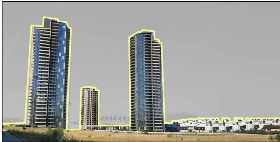
Figure 4.11. Icon, Incek Edited by the author on Google Earth Street Views dated 7.2019.
