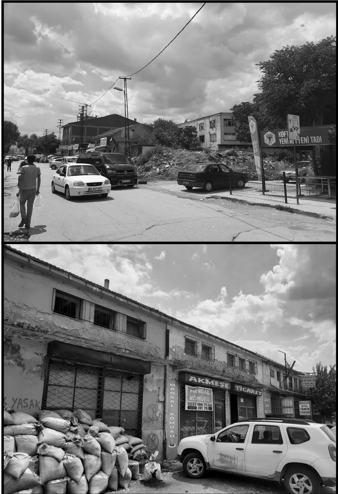
Figure 4.3 Ruined and dilapidated buildings that give a negative image of the place.
