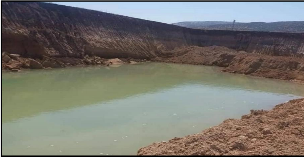
Figure 4.34: Pazarcık State Hospital Construction Foundation Excavation
