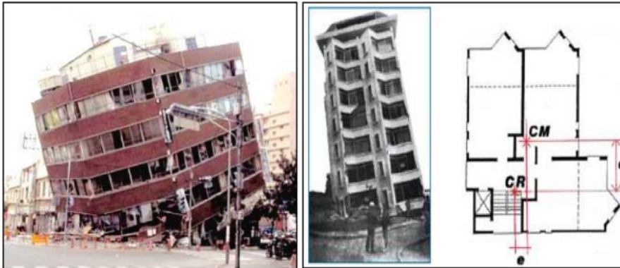
Figure 3.16: Collapse due to Torsion
