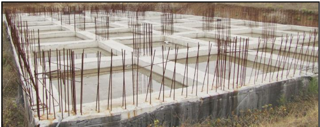
Figure 4.54: Unfinished Foundation Construction
