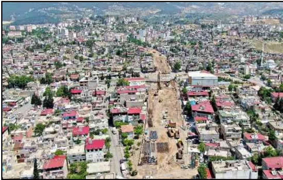
Figure 4.44: An Example of Crossover Road Construction
