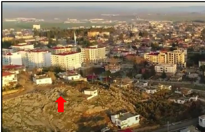
Figure 4.48: Constructions on Infill Ground
