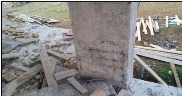
Figure 4.52: The Building with the Concrete Pouring Work
