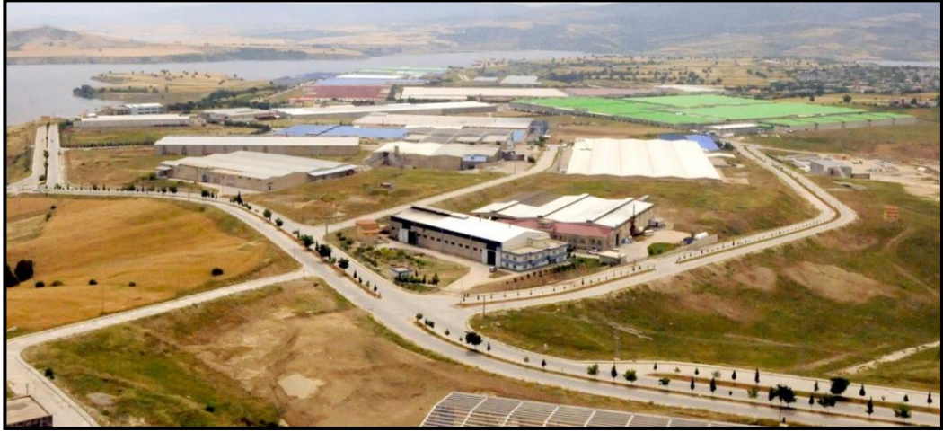
Figure 4.41: Industrial Structures around the Osmaniye Ring Road
