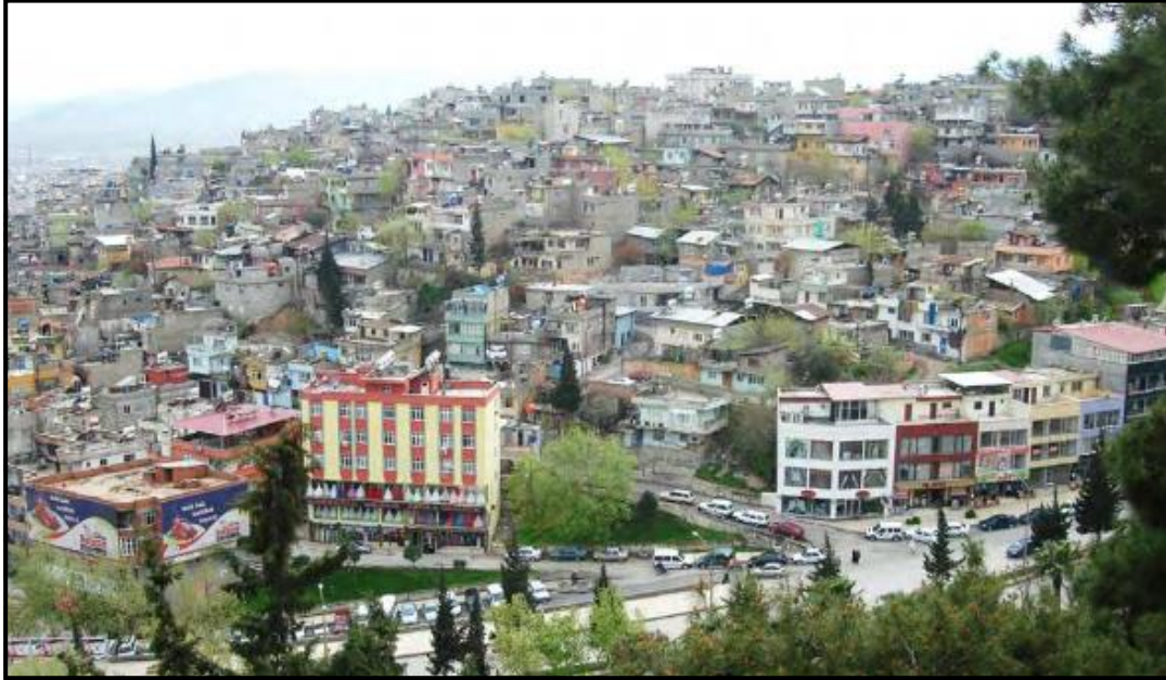
Figure 4.28: Irregular Construction View in Kahramanmaraş
