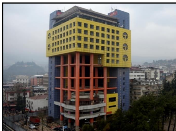
Figure 4.50: Private Administration Business Center Building with Various Seismic Design Faults
