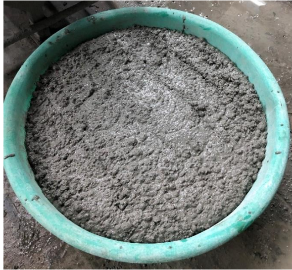
Figure 4.5 Concrete Mix in the Plastic Basin
