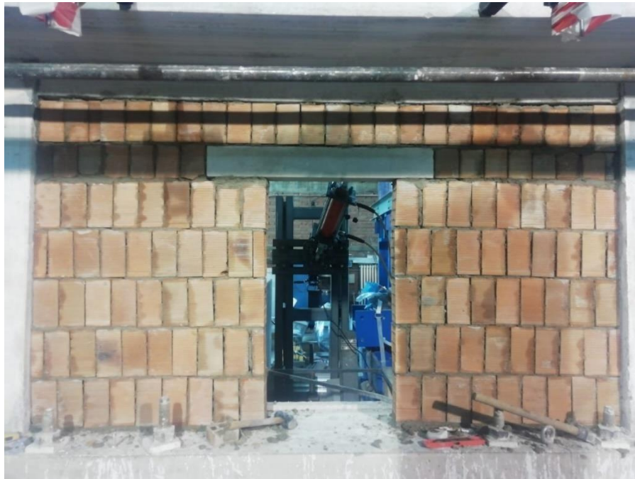
Figure 2.23. Built WBVD Without Plaster on it
