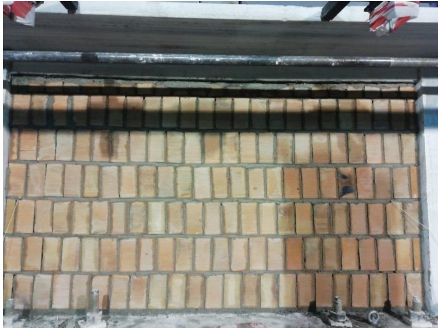
Figure 2.11. Built WBVN1 Without Plaster on it
