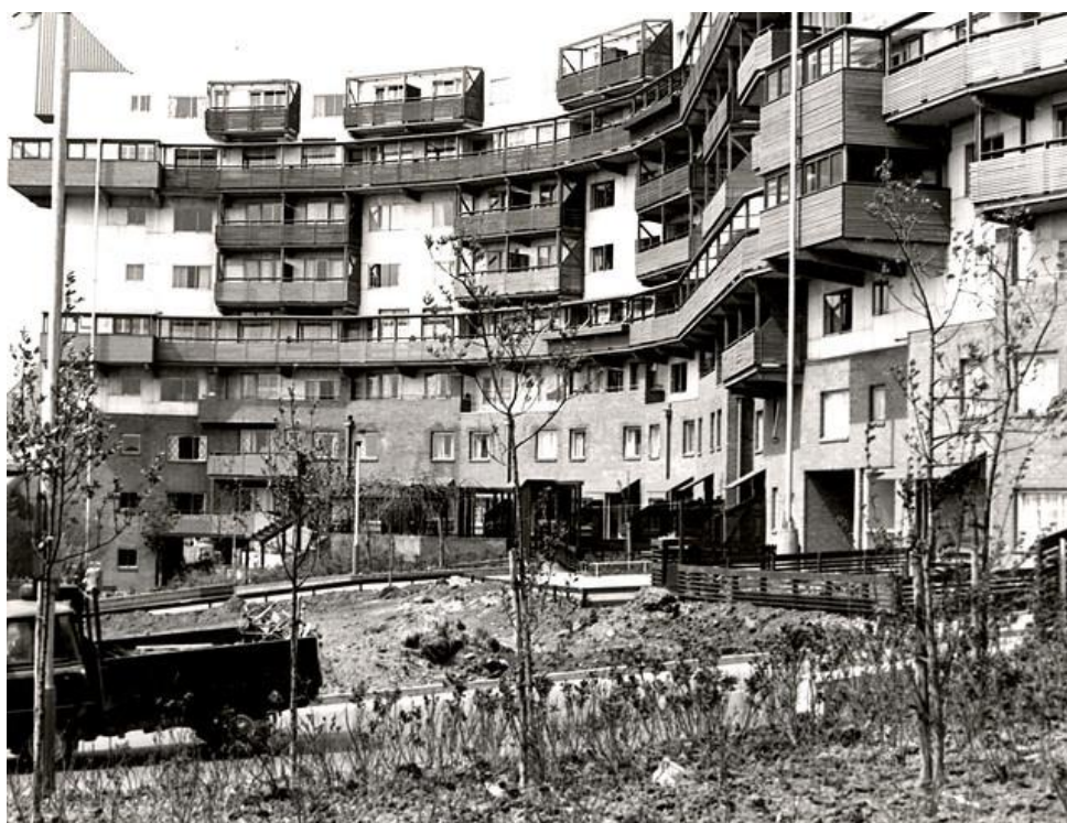
Figure 13: An image of the Byker Wall project in Newcastle showing the individual modifications and projections on parts of the façade made by inhabitants. Image source: Newcastle Libraries, Byker Wall Byker City Engineers, 1974, https://www.flickr.com/photos/39821974@N06/4078269651/ .
