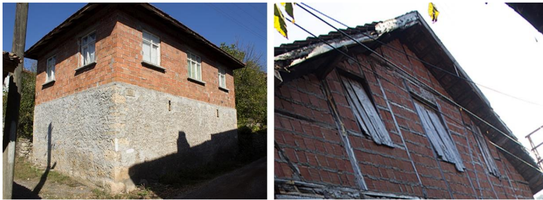
Figure 3.40. Hacilarobası, a building with brick masonry on the upper floor (left) and reuse of timber with brick infill (right)
