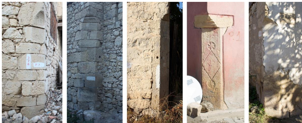
Figure 3.36. Hacilarobası, examples of chamfered corners of the traditional buildings
