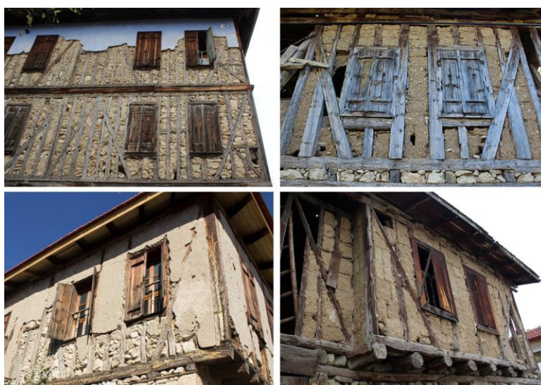
Figure 3.38. Hacilarobası, timber frame structures with rubble stone and mudbrick infills
