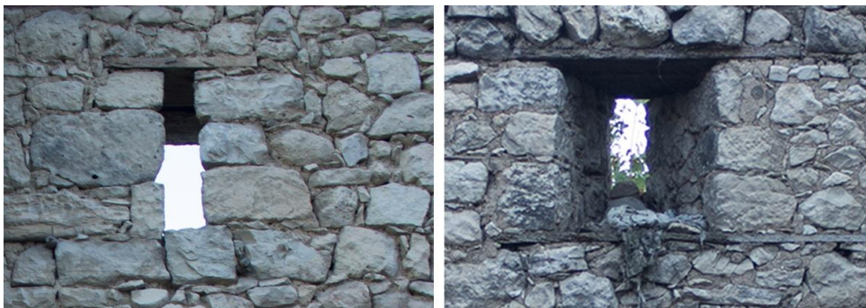
Figure 3.37. Hacilarobası, a typical opening as seen from outside and inside
