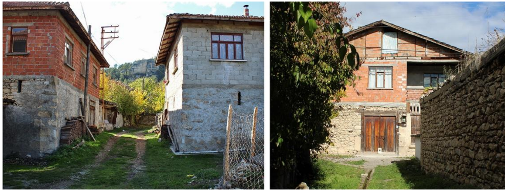
Figure 4.19. Hacilarobası, examples of reconstruction of the upper floors with new construction techniques
