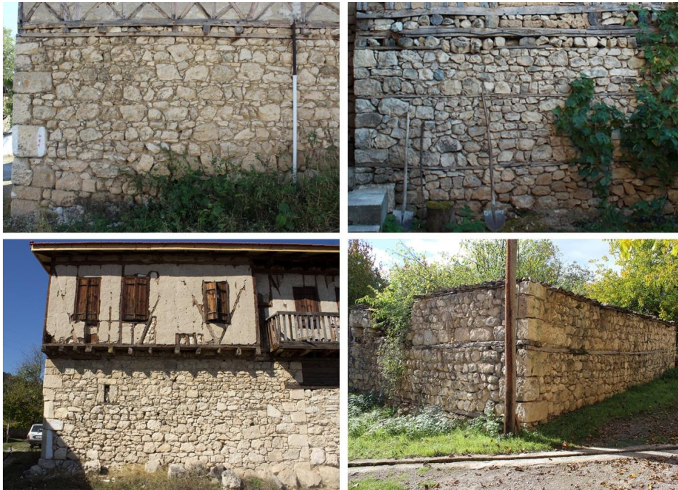
Figure 3.35. Hacilarobası, stone masonry walls
