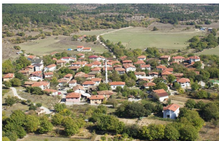
Figure 3.39. Hacilarobası, roof coverings
