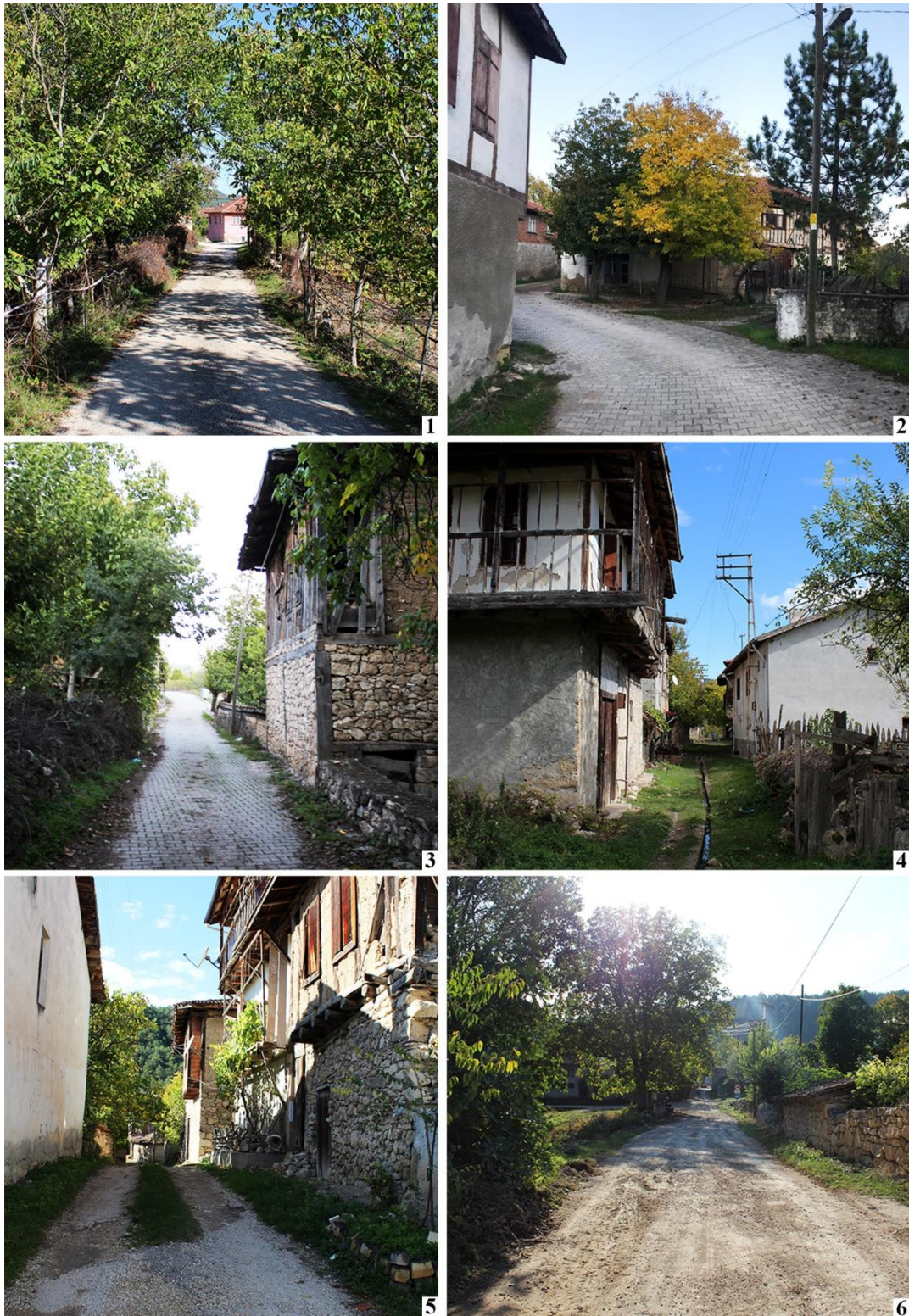
Figure 3.19. Hacilarobasi, pavement types: (1) asphalt; (2 and 3) cobble; (4) water channel in the street; (5) asphalt pavement in a deteriorated state; (6) dirt
