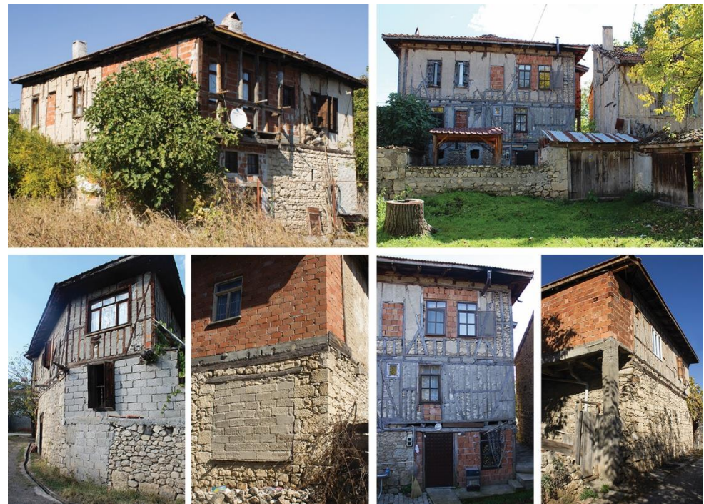
Figure 4.21. Hacilarobası, examples of interventions incompatible with the vernacular fabric
