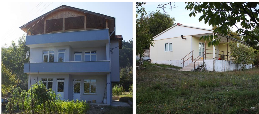
Figure 3.41. Hacilarobası, reinforced concrete (left) and prefabricated buildings (right)
