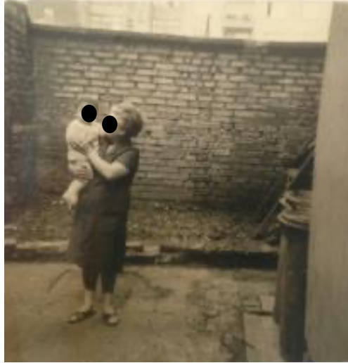
Figure 6.1: Nur photographed her neighbor in the backyard of their building in Duisburg. Circa 1973. Source: Nur's album
