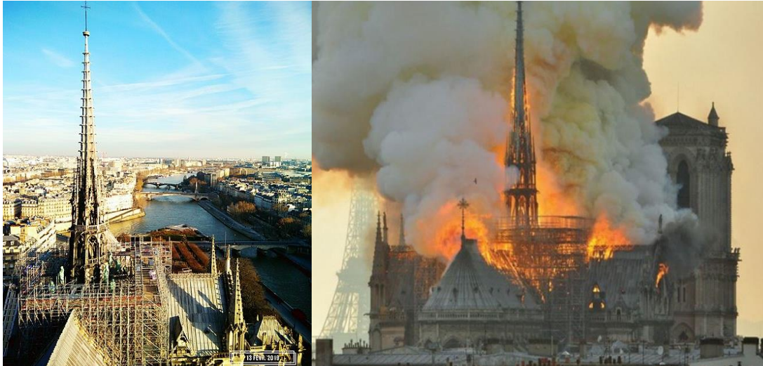
Figure 6.14. (Left) The spire of Notre-Dame under restoration, before the fire of 2019. (Source: https://en.wikipedia.org/wiki/File:Vue_de_la_fl%C3%A8che_depuis_les_tours.jpg ) (Right) The spire of the Notre-Dame Cathedral during the early stages of the 2019 fire. (Source: Wikimedia Commons)
