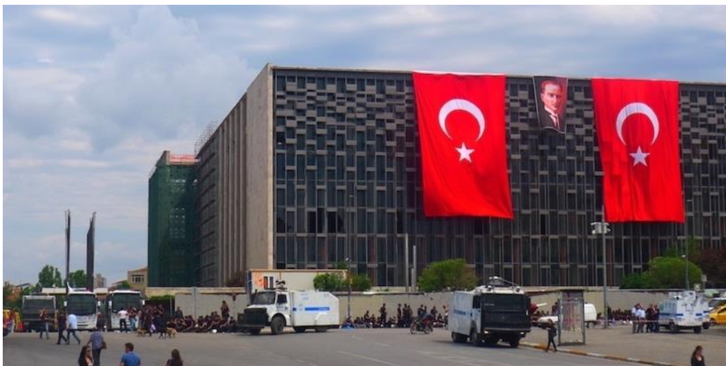
Figure 274 AKM turned into a police station after Taksim Square clearance. Mid-June.
