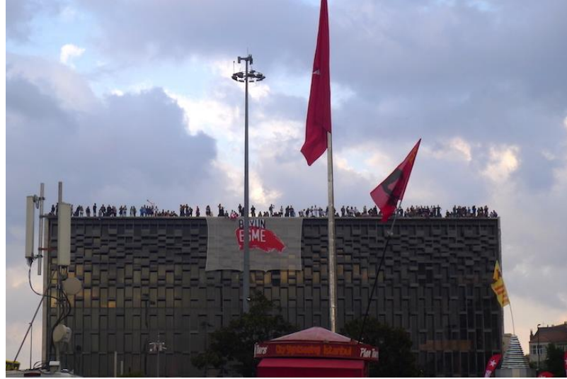
Figure 220 First banner on the AKM façade. 2013, June 2.
