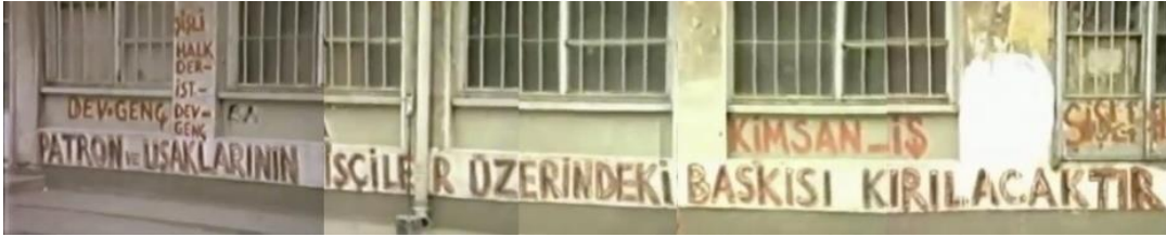
Figure 44 Montage of still frames of the comedy film Köşeyi Dönen Adam (The Man Who Gets Rich) (Yılmaz, 1978). Writing at the bottom: “the oppression of the boss and his servants over the workers will be broken”.
