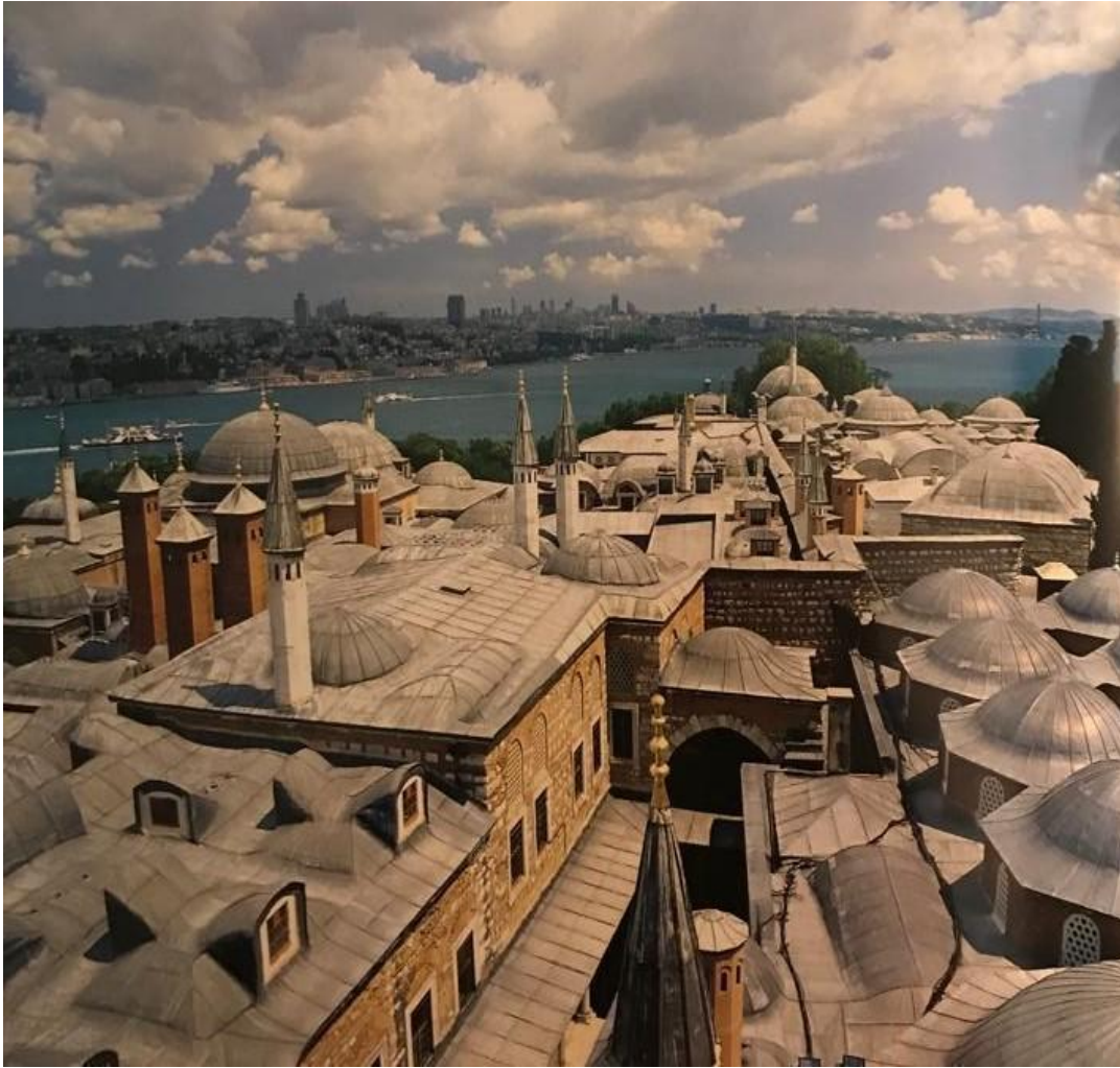
Figure 8.77 Lead domes of Topkapı Palace Harem Section.
