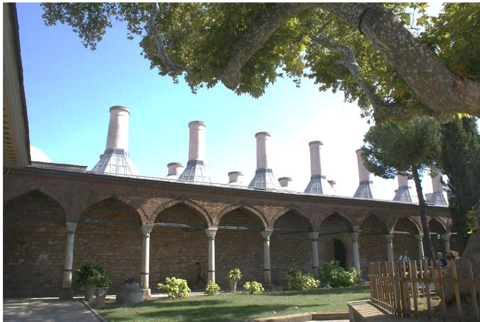
Figure 8.76 Brick, marble and lead materials on the Kitchen structures. Source: Filiz Kölmek, “Kitchen structures” (photo, 2020).
