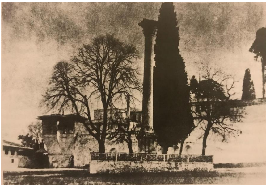
Figure 8.100 Photograph dated 1852 shows the third court’s hanging garden, some of the mansions that have disappeared today, and the Column of the Goths in front of it. Source: Architecture, Ceremonial and Power, Topkapı Palace in the 15 th and 16 th Centuries , “Hanging garden,” (photo, 1852), 251.
