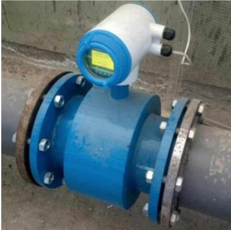
Figure 3.4 Magnetic Flowmeter
