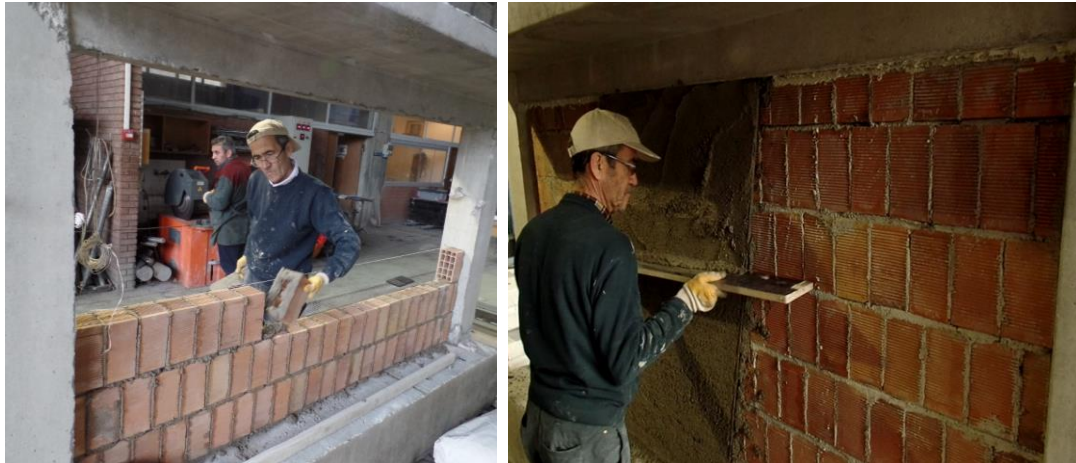
Figure 3.10. Construction of HCB infilled frame with plaster
