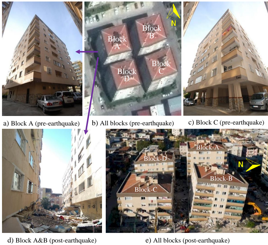
Figure 1.5. Barış apartment complex in İzmir, 2020 Samos EQ ( M_w=6.9 )
