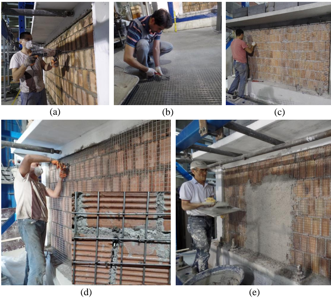
Figure 3.11. Construction sequence of CBMR specimen
