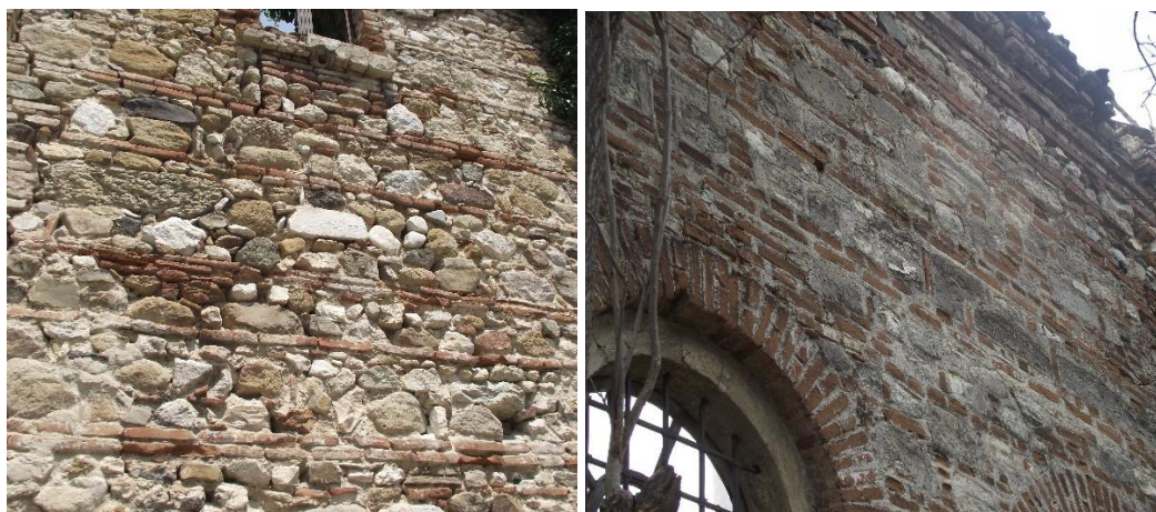
Figure 4.2. Alternating courses of stone and brick technique as seen in Aydınpınar, Hagios Ioannes (left); Dereköy, Hagia Paraskevi (right) (2021)
