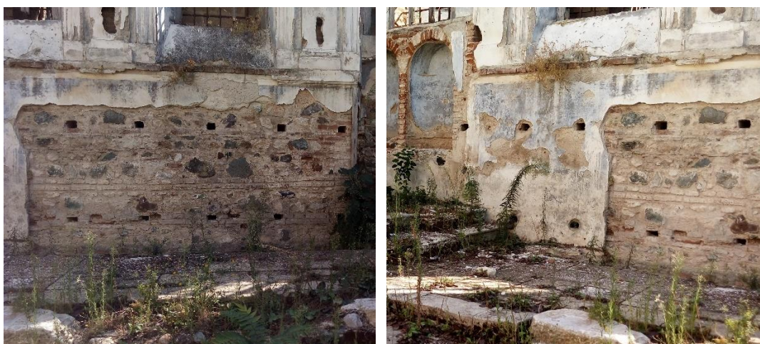
Figure 4.3. Dereköy, Hagia Paraskevi, perforated structure on the south wall of the naos (2021)
