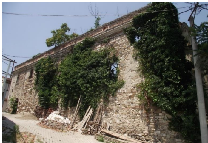
Figure 3.35. Aydın, Hagios Ioannes, south façade (2021)
