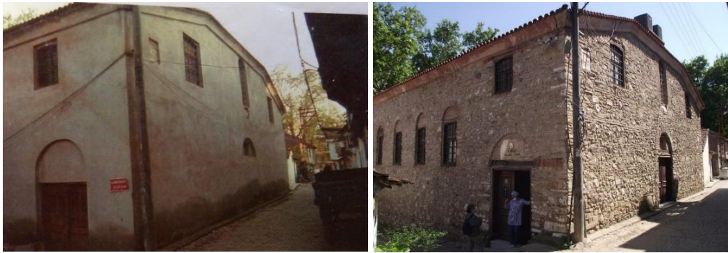
Figure 3.68. Tirilye, Panagia Metropolis, northeast façade (above) (Mudanya Municipality Archive, 2003); view from the north before restoration (below left) (BKVKBK, 2001); view from the north (below right) (2021)
