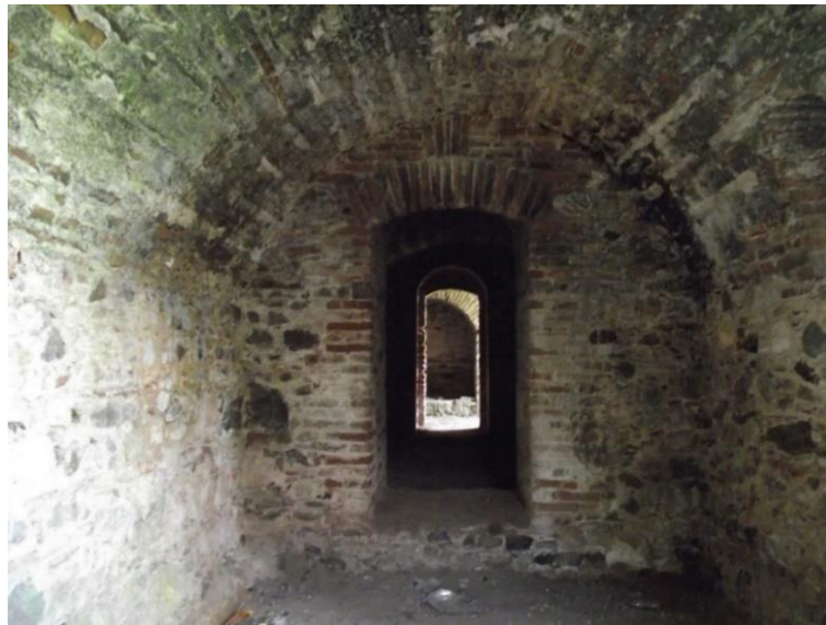
Figure 3.47. Dereköy, Hagia Paraskevi, basement (2021)
