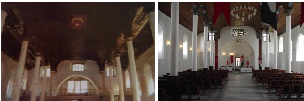
Figure 3.66. Tirilye, Panagia Metropolis, apse and ceiling as seen from the naos, before restoration (left) (BKVKBK, 2001); apse as seen from the narthex (right) (2021)
