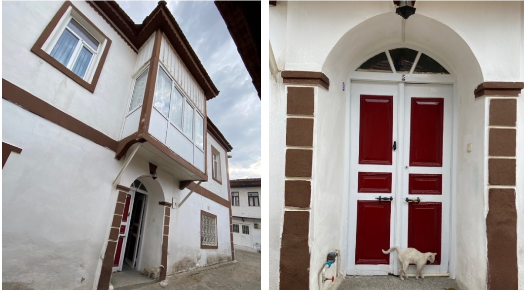
Figure 72 Case #11 House - Street Facade
