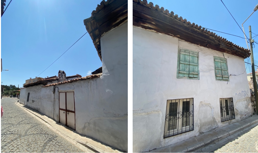
Figure 59 Case #9 House - Street Facade
