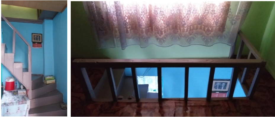
Figure 82 Case #12 House - Staircase
