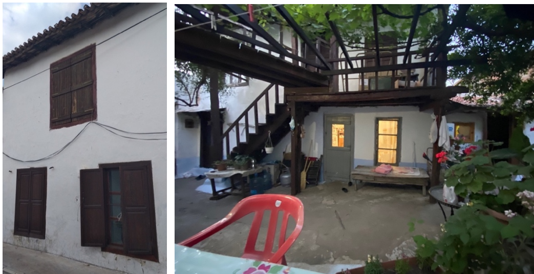
Figure 35 Case #4 House - Main Building - Street Facade and Courtyard Facade
