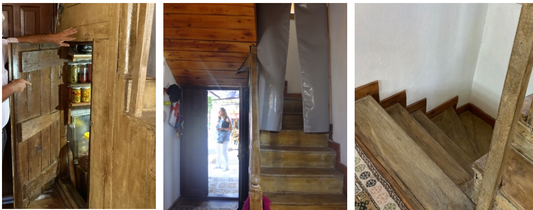
Figure 25 Case #2 House - Staircase
