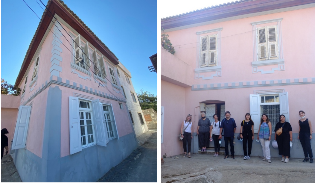
Figure 29 Case #3 House - Street Facade
