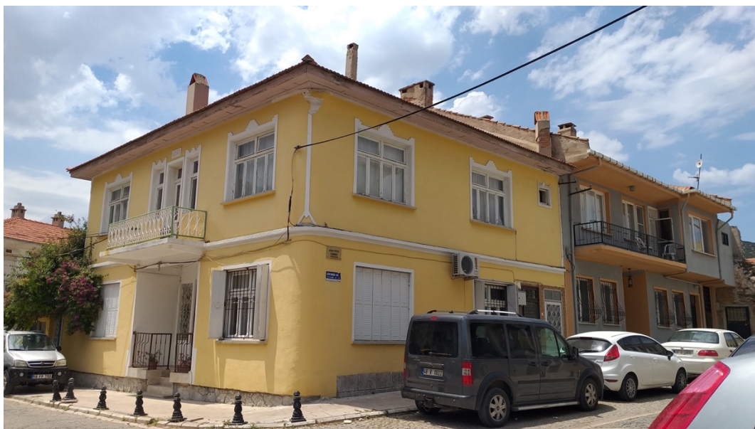
Figure 38 Case #5 House - Street Facade
