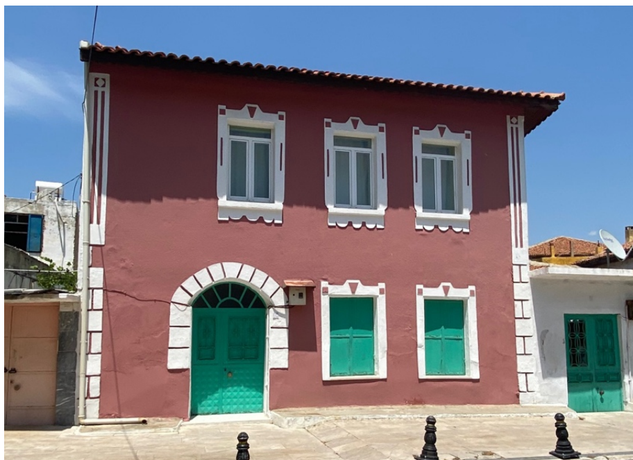
Figure 78 Case #12 House - Street Facade
