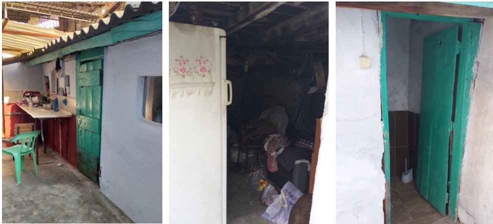
Figure 63 Case #9 House - Service Building
