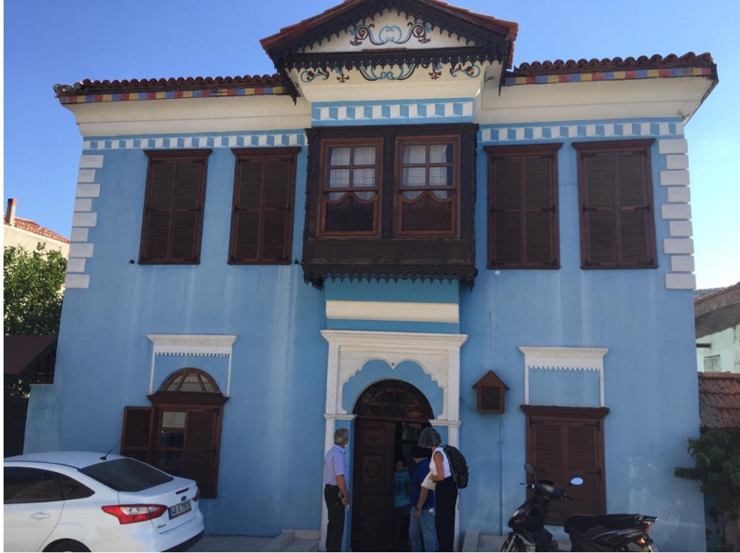
Figure 13 Case #1 House - Street Facade
