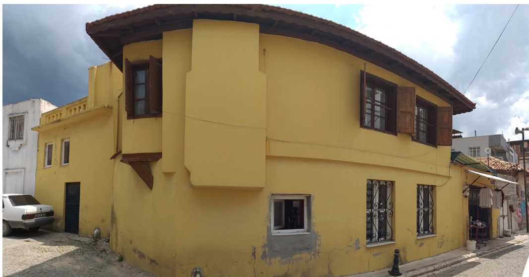
Figure 101 Case #16 House - Street Facade
