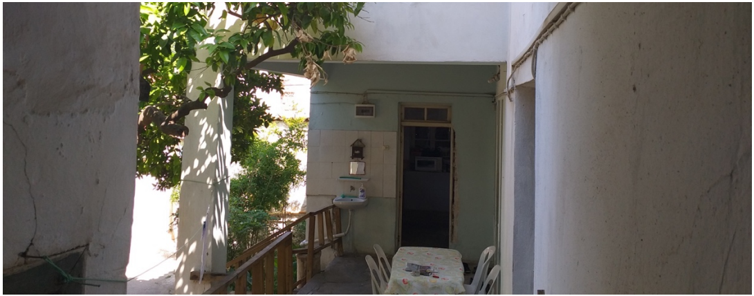
Figure 95 Case #15 House - Space Addition (Kitchen)
