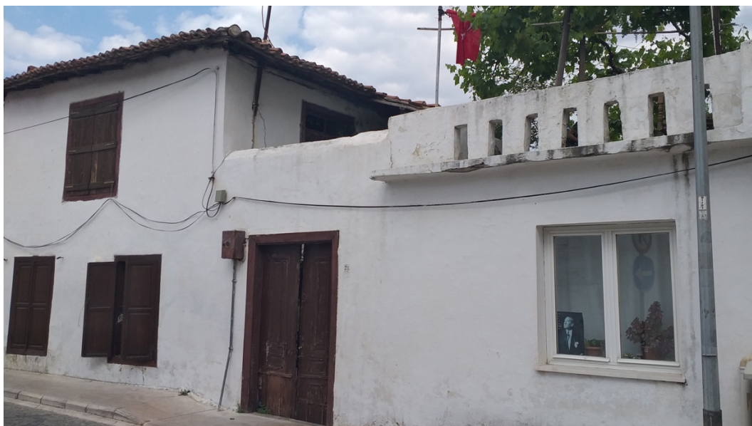
Figure 32 Case #4 House - Street Facade
