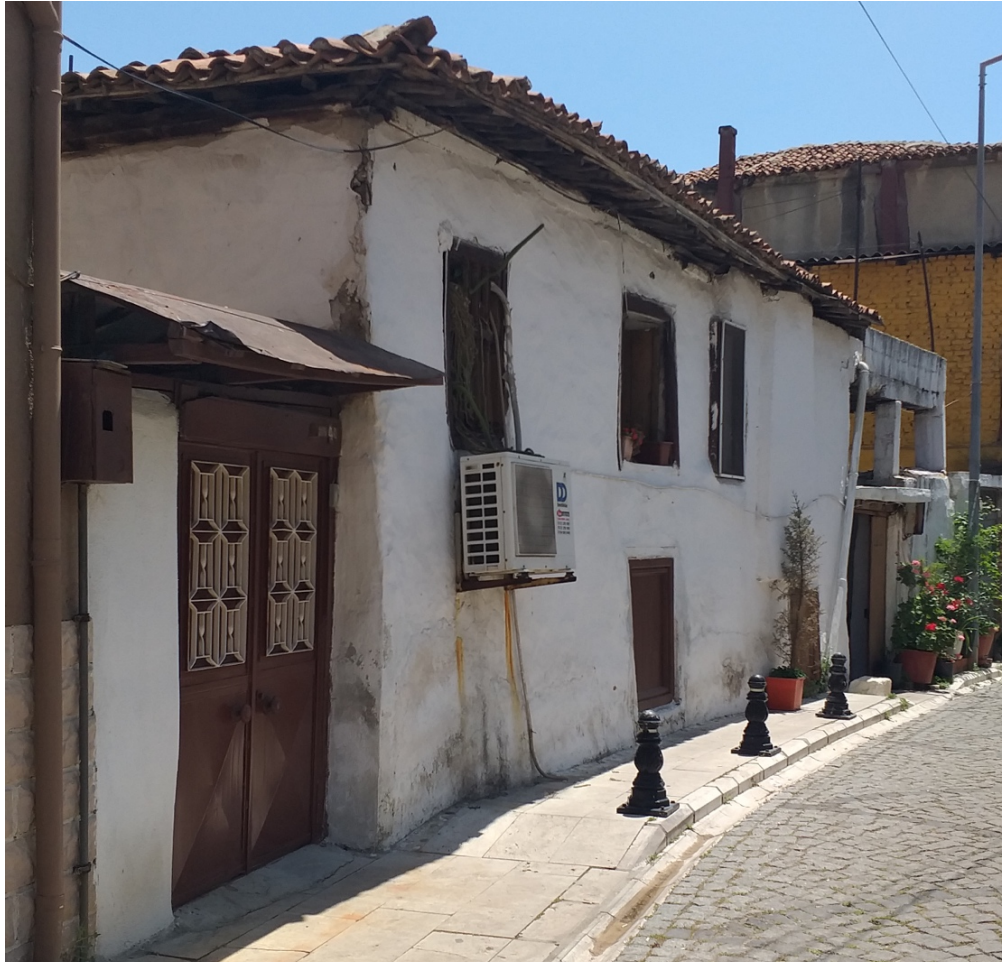
Figure 44 Case #6 House - Street Facade
