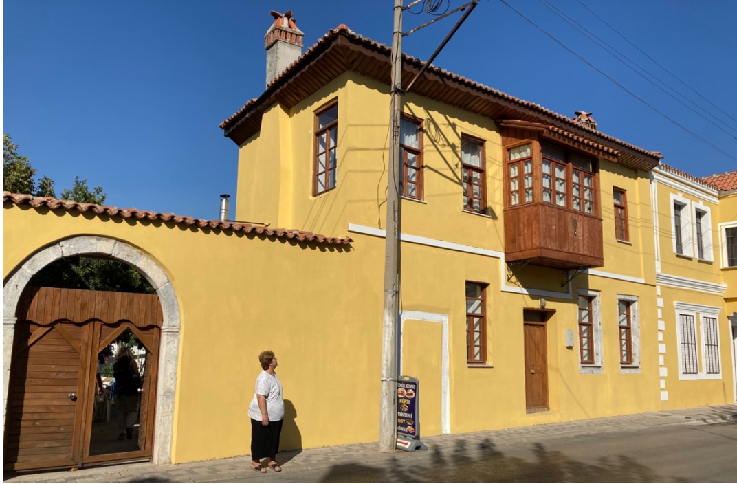
Figure 21 Case #2 House - Street Facade
