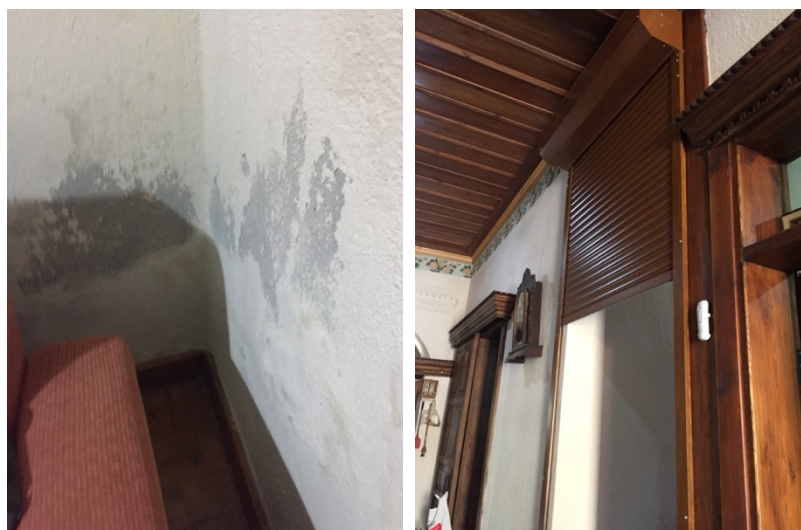
Figure 20 Case #1 House - Ground Floor Walls and Shutter
