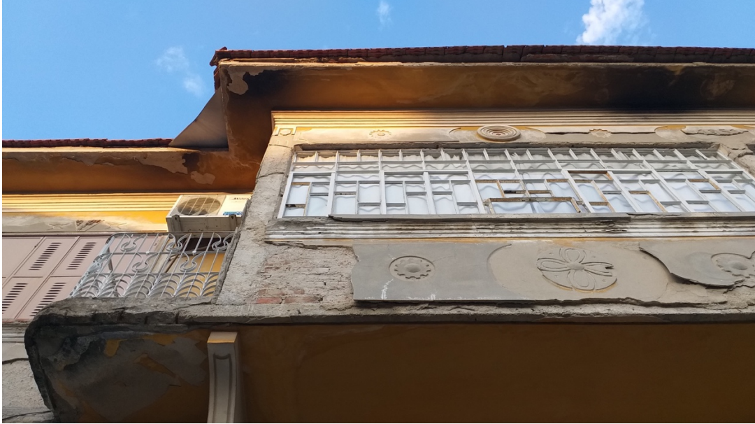
Figure 64 Case #10 House - Street Facade
