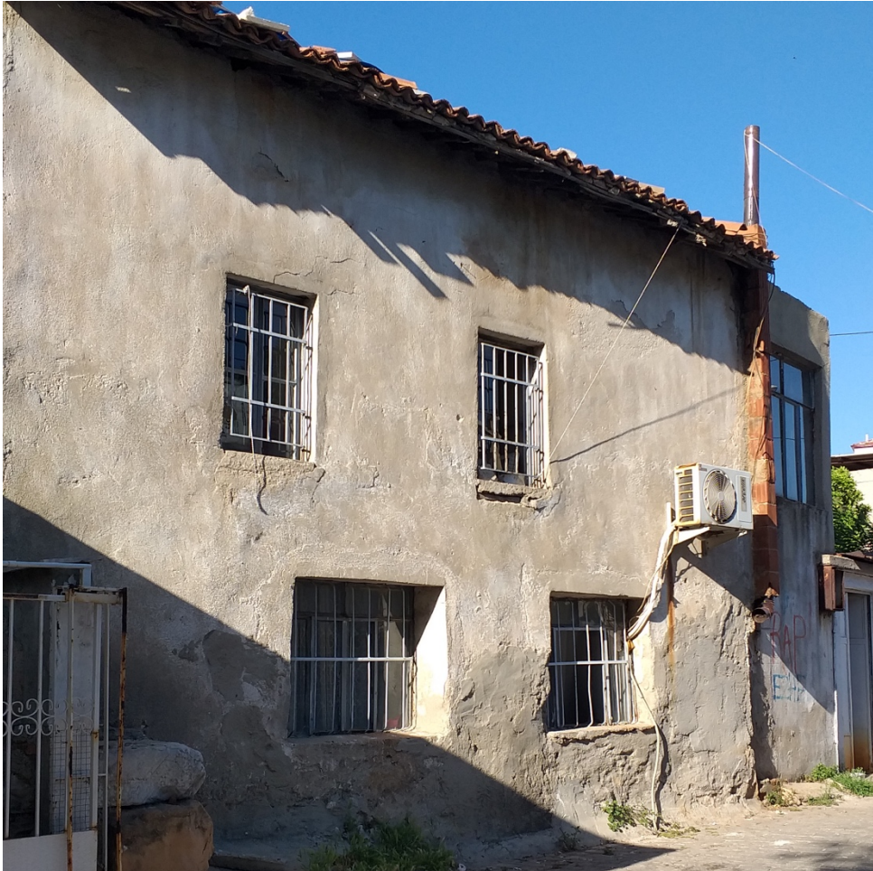
Figure 89 Case #14 House - Street Facade
