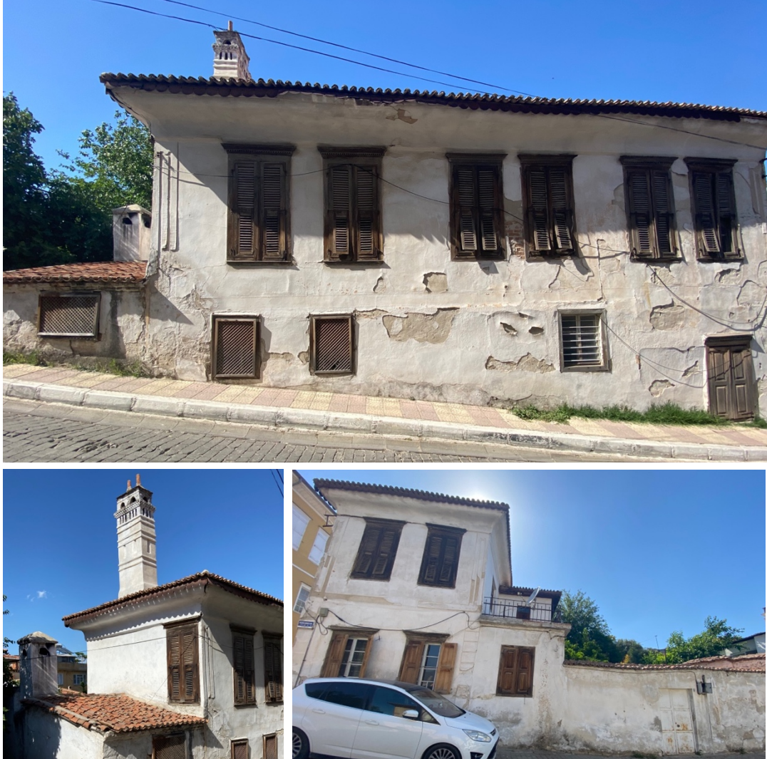
Figure 93 Case #15 House - Street Facade
