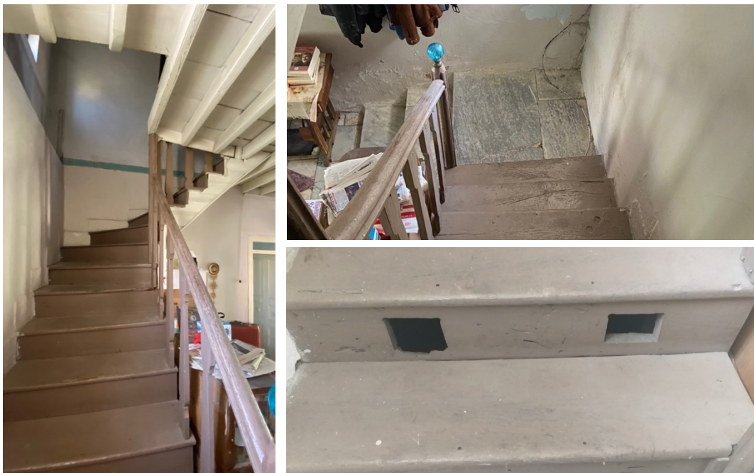
Figure 97 Case #15 House - Staircase
