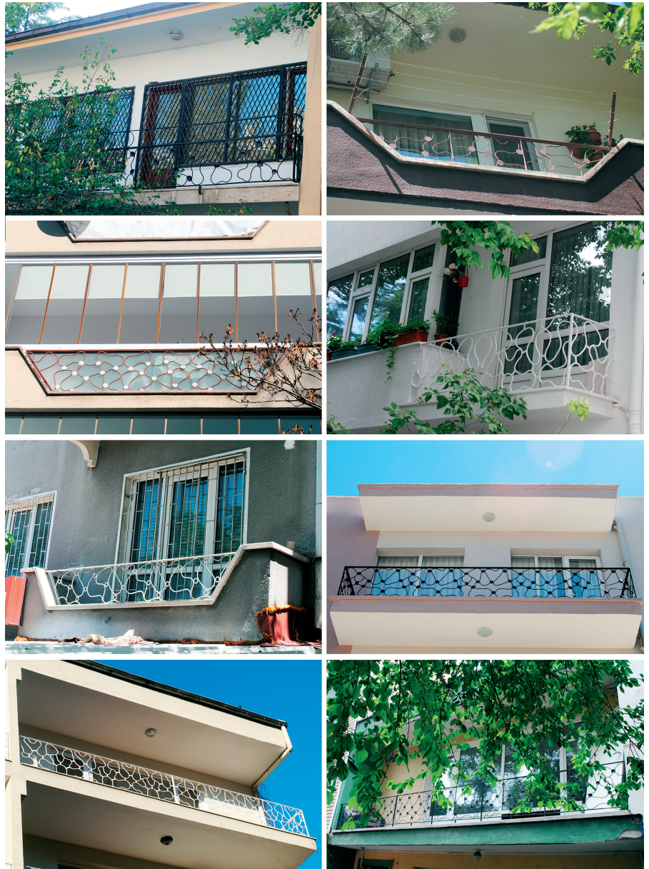
Figure 7. Similar balcony balustrade samples dispersed across Çankaya District (Tuna Ultav archive)
