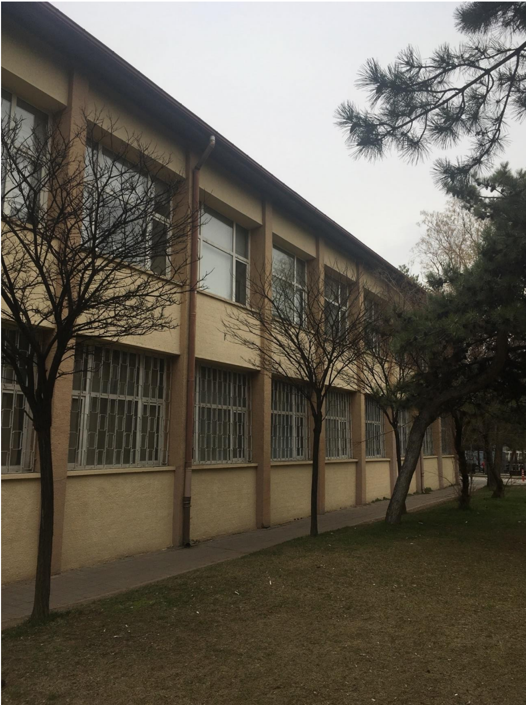
Photograph 8. The building of ELT department which is currently used since 1980s
