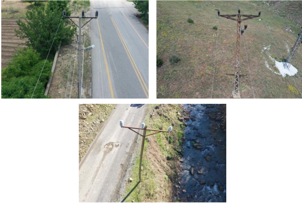
Figure 18. Concrete, Steel, and Wooden Electricity Pole Images
