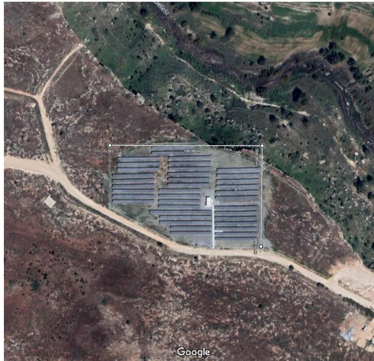
Figure 4.2: METU NCC Solar PV areas from google maps
