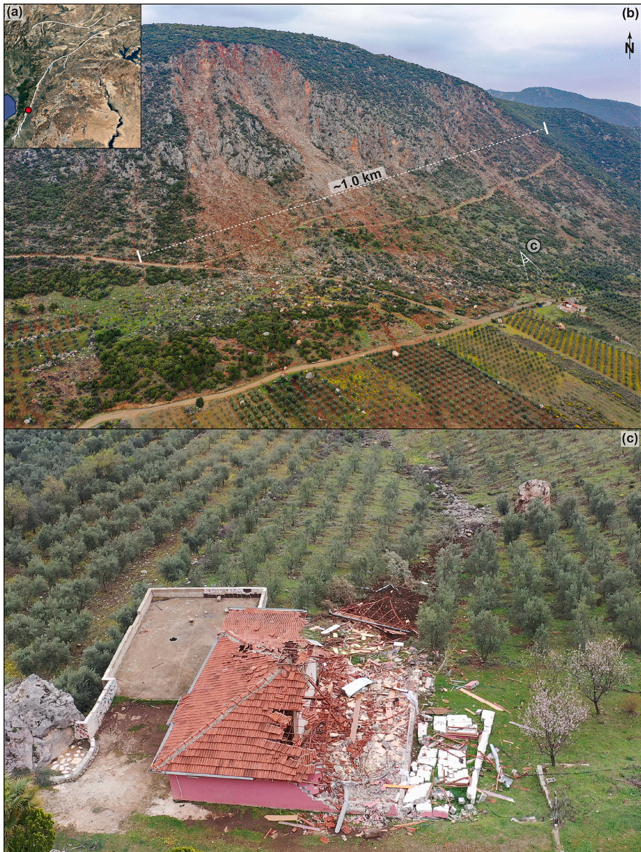
Fig. 10. Drone images showing an area affected by rock falls (lat: 36.67°, lon: 36.43°) near Kırıkhan, Hatay. The red point in panel (a) shows the landslide location. Panels (b) and (c) show the entire hillslopes exposed to rock falls and a house destroyed by a rock fall, respectively. The width of the hillslope was indicated in panel (b) as a bar scale. The viewing angle of panel (c) was indicated in panel (b). (For interpretation of the references to colour in this figure legend, the reader is referred to the web version of this article.)
