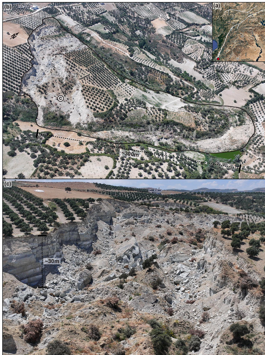
Fig. 12. Aerial photos showing the translational slide (lat: 36.16°, lon: 36.22°) triggered near Altınözü, Hatay. The red point in panel (a) shows the landslide location. Panels (c) and (d) show the entire landslide body and the crown of the landslide, respectively. The viewing angle of panel (c) was indicated in panel (b). (For interpretation of the references to colour in this figure legend, the reader is referred to the web version of this article.)
