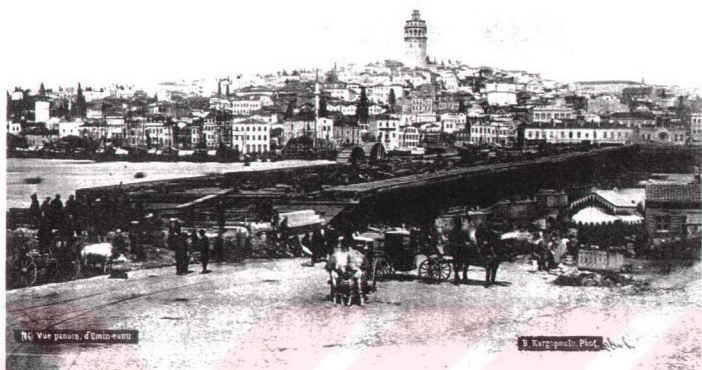
Fig. 55.1. The construction of the second Galata Bridge, photography by Kargopulo, 1875 (Yerasimos, M., 1990)
