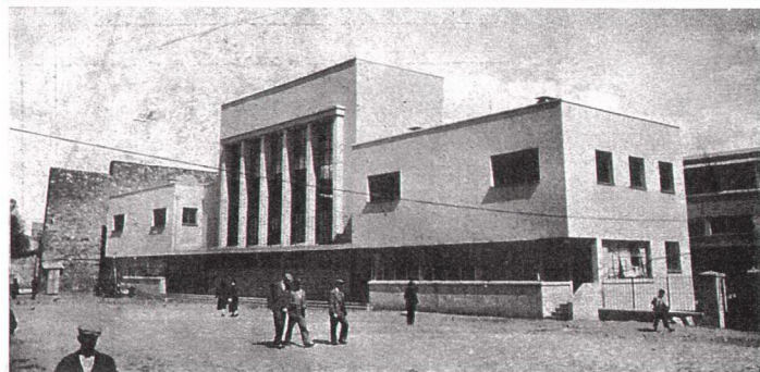
Fig. 70.2. New Fruit Exchange, from the sea and the road construction early 1930s, photograph, 1934 (after, Arkitekt) The wall at the back is the fire-wall of the former wharf of building constructions.
