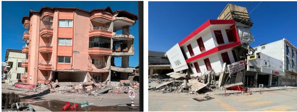
Figure 5. Failures due to the soft story on the ground floor from Antakya, Hatay
