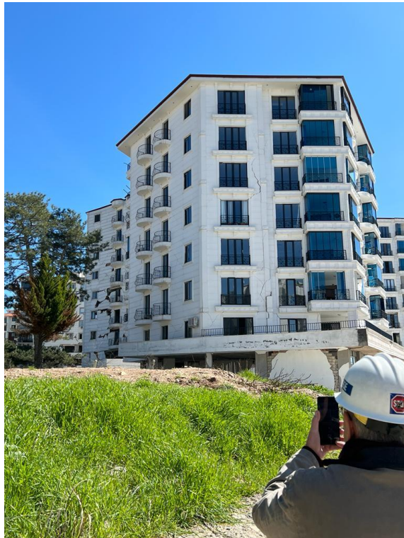
Figure 8. Severely damaged hotel building with plan irregularity from Adiyaman
