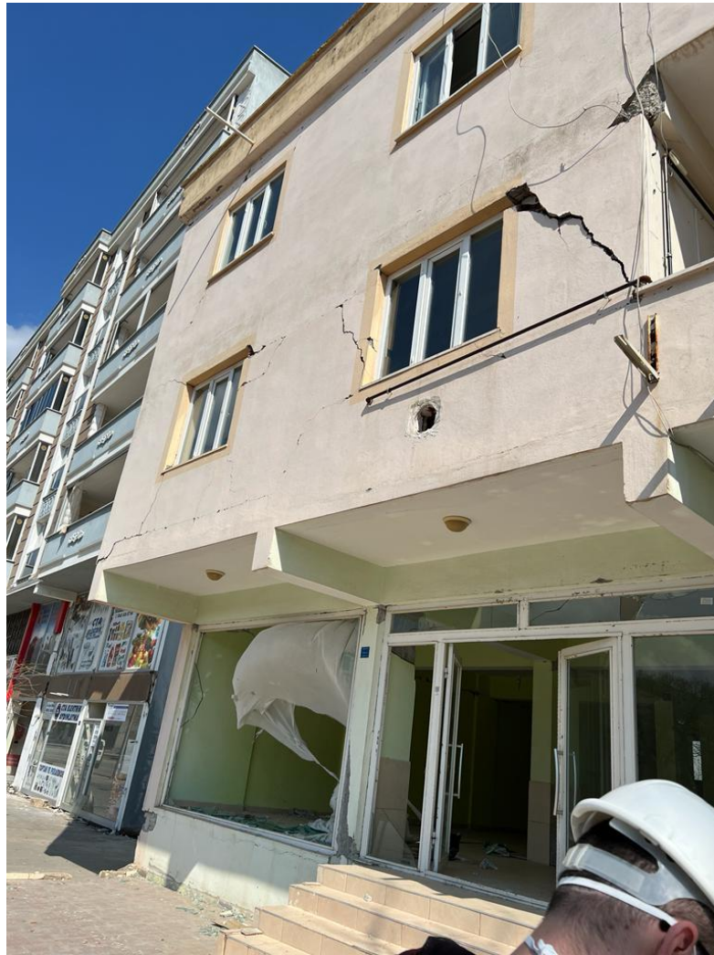
Figure 3. A real-life example of excessive overhangs from Turkoglu, Kahramanmaraş
