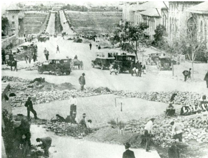
Figure 15: A photograph from 1925 showing the work on laying cobblestones in Hakimiyet-i Milliye Square.
