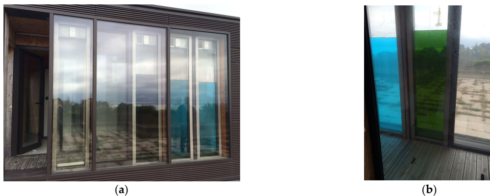
Figure 12. Biofaçade SymbIO 2 Box prototype; (a) Biofaçade from the exterior view, (b) Biofaçade inside the SymbIO 2 Box, created at AlgoSolis, GEPEA in Saint Nazaire, France, developed by XTU Architects, scientifically equipped by the GEPEA, inauguration 2015. Images: Natasha Heil.
