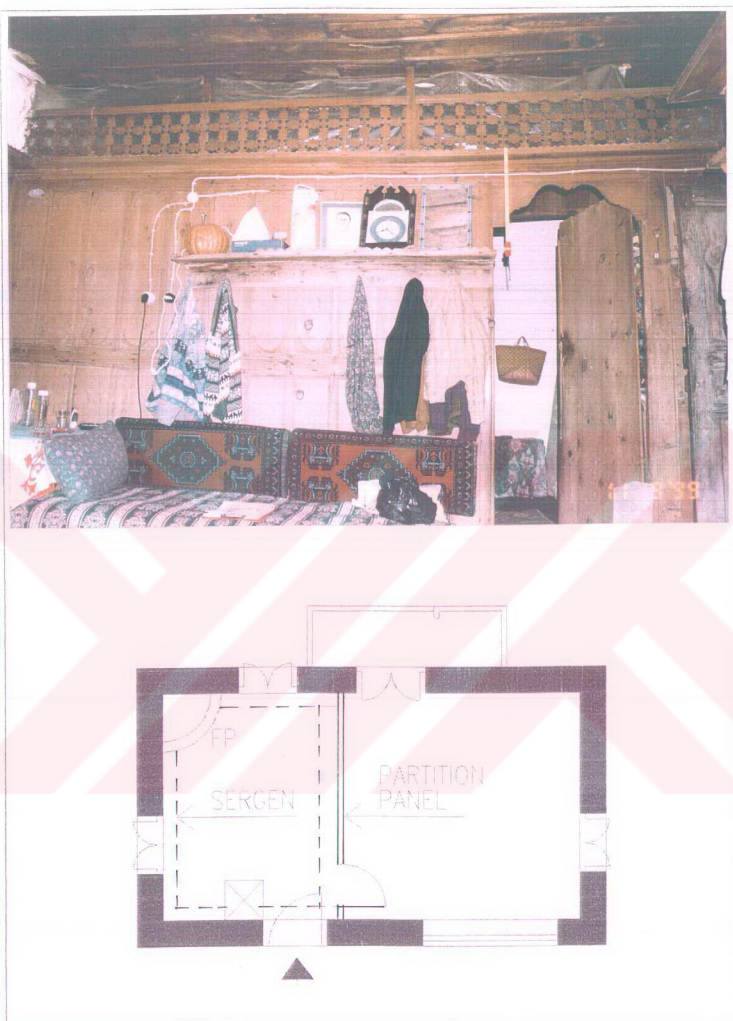
Figure 4.8: Partition Panels Dividing the Main Space (F.9.3)
