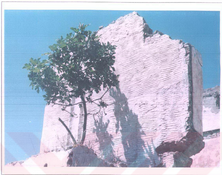
Figure 3.54 : Facade Textures by Using Nailing ( çivileme ) Technique
