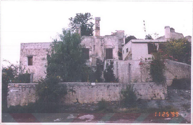
Figure 4.41 : Elongation of Chimney (F.4.3.) and Additional Building (F.4.4)
