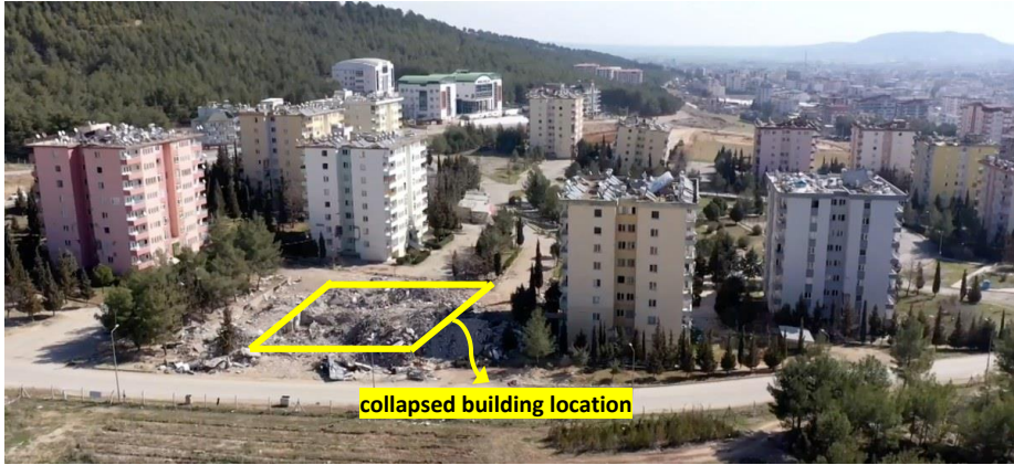
Figure 1.1: Block of similar RC constructions in Adiyaman after the 2023 earthquakes: one collapsed, the others experienced various degrees of damage
