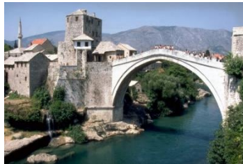
Figure 2.36. Conservation of Mostar Old Town, Bosnia-Herzegovina Source: archnet.org
