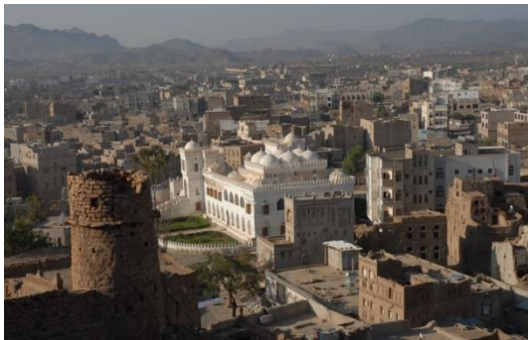
Figures 3.29. Restoration of Amiriya Complex, Rada, Yemen. 2007. Source: Archnet.org
