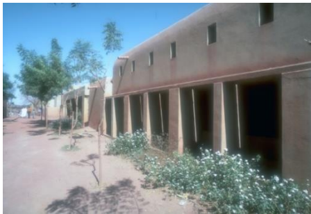
Figure 3.11. Mopti Medical Centre, Mali. 1980 Source: Archnet.org
