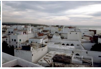
Figure 2.56. Rehabilitation of Asilah, Morocco Source: archnet.org
