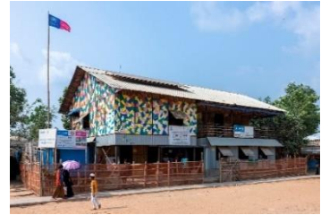
Figure 2.134. Community Spaces in Rohingya Refugee Response, Bangladesh Source: archnet.org
