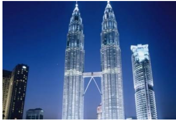
Figure 2.97. Petronas Office Towers, Malaysia Source: archnet.org
