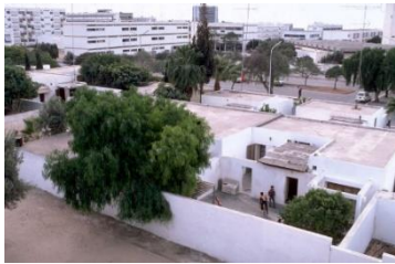
Figure 2.12. Courtyard Houses, Morocco Source: archnet.org
