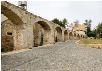
Figure 2.104. Rehabilitation of the Walled City, Cyprus Source: archnet.org
