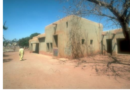
Figure 3.12. Mopti Medical Centre, Mali. 1980 Source: Archnet.org
