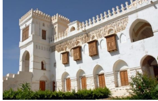
Figures 3.28. Restoration of Amiriya Complex, Rada, Yemen. 2007. Source: Archnet.org
