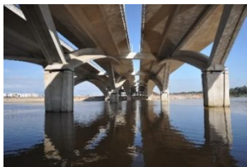
Figure 2.115. Hassan II Bridge, Morocco Source: archnet.org
