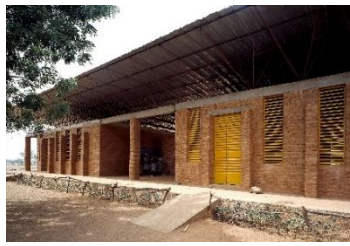
Figure 2.98. Primary School, Burkina Faso Source: archnet.org
