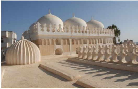
Figures 3.27. Restoration of Amiriya Complex, Rada, Yemen. 2007. Source: Archnet.org
