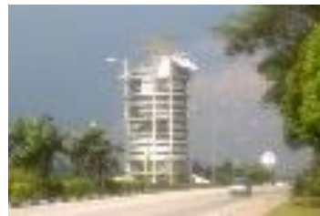
Figure 2.75. Menara Mesiniaga, Malaysia Source: archnet.org
