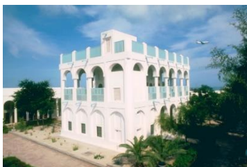
Figure 2.19. National Museum, Qatar Source: archnet.org
