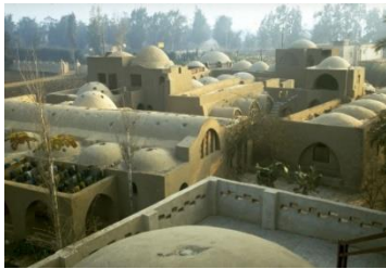
Figure 2.30. Ramses Wissa Wassef Arts Centre, Egypt Source: archnet.org
