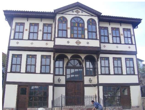
Figure 4.23. Post-intervention view of east side facade (Author, 2013)
