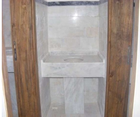
Figure 4.12. A4, alteration of bathrooms I (taken from the Taraklı Municipality, 2013)
