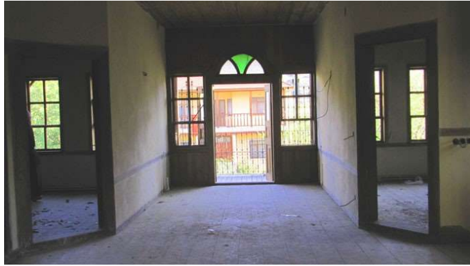
Figure 3.72. Post-intervention of sofa on second floor after its transformation (Author, 2013)
