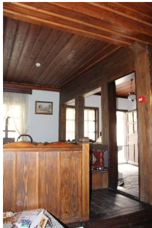
Figure 4.39. Post-intervention views of GPOI08 (Author, 2013)
