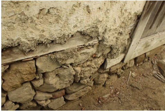
Figure 2.12. Stone foundation of Ezancılar house (Author, 2016)
