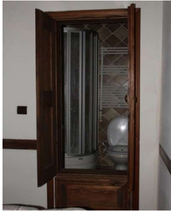
Figure 3.46. Post-intervention view of FPOI03 (bathroom) (Author, 2016)
