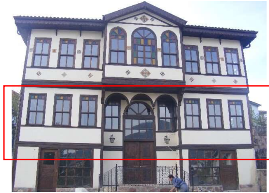
Figure 4.8. A1. Post-intervention view of east side facade that show the alterations of windows at first floor (Author, 2013)
