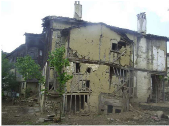
Figure 3.54. Pre-intervention view of Hacı Rıfatlar house, east facade (Özkan, 2008, p.123)
