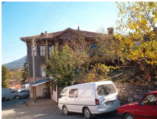
Figure 4.5. Pre-intervention view of north side facade (taken from the Taraklı Municipality, 2013)
