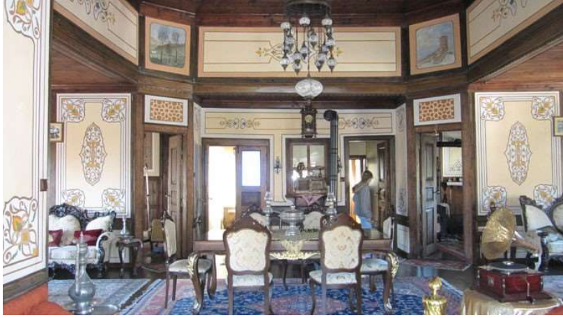
Figure 2.24. Kalemîşi ornamentation on wall of 2.nd floor sofa of Kadirler house after its transformation (Author, 2013)
