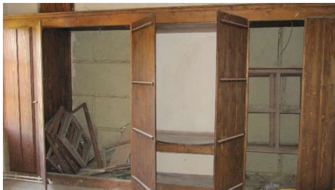
Figure 3.74. Post intervention of rooms on second floor after its taransformation (Author, 2013)
