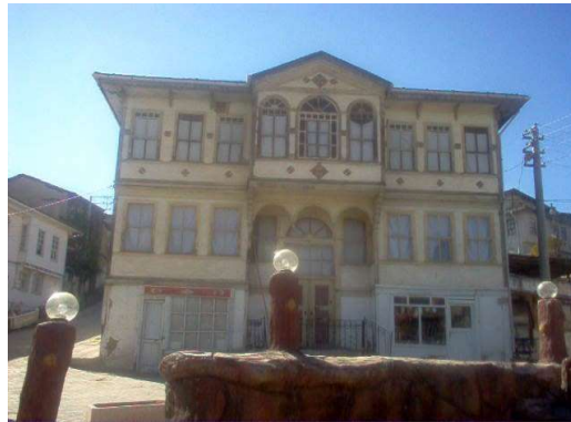
Figure 3.4. Pre-intervention view of Kadirler house, east facade (taken from the Taraklı Municipality, 2013)
