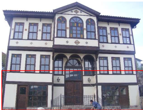
Figure 4.2. Post-intervention view of east side facade that show the alterations of entrance staircase and alterations of shop windows and doors at ground floor (Author, 2013)
