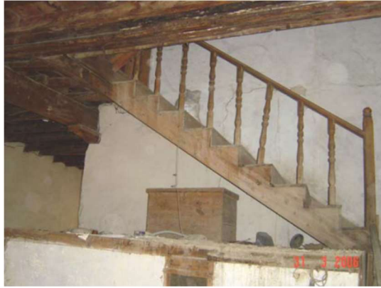
Figure 4.60. Pre-intervention view of the GPOI03 that indicate the G.R1 (Selçuk, 2008, p.104)
