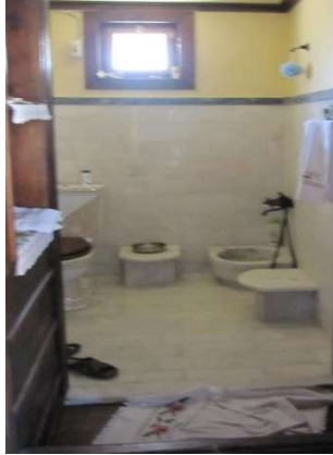
Figure 4.20. S.A4, Alteration of a bathroom (Author, 2013)
