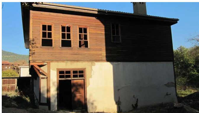
Figure 3.63. Post-intervention view of Hac1 Rıfatlar house, west facade (Author, 2013)
