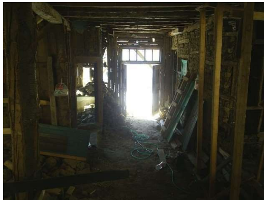
Figure 4.42. Pre-intervention views of GPOI06 (taken from the Taraklı Municipality, 2013)
