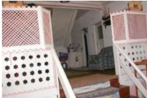
Figure 4.79. Pre-intervention view of the entrance staircase at right side (Çetin, 2006, p.548)
