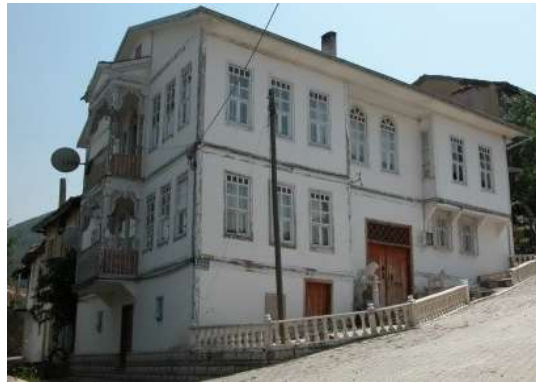
Figure 3.77. Pre-intervention view of Çakırlar house, north-east facade (Çetin, 2006, p.546)
