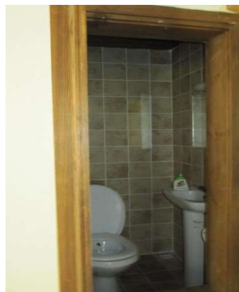
Figure 3.40. WC solution in a bedroom of ground floor, GPOI07 (Author, 2016)
