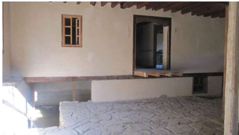
Figure 3.68. View of basement floor and mezzanine (first) floor from the main entrance (Author, 2013)
