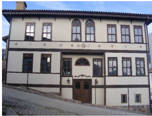
Figure 4.32. Post-intervention view of south facade (Author, 2013)
