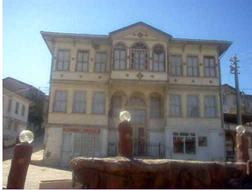
Figure 4.3. Pre-intervention view of east side facade that show the alterations of entrance staircase and alterations of shop windows and doors at ground floor (taken from the Taraklı Municipality, 2013)
