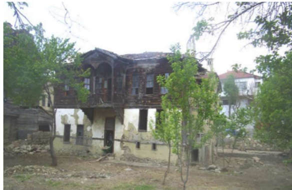
Figure 3.52. Pre intervention view of Hacı Rıfatlar house, south facade (Özkan, 2008, p.121)
