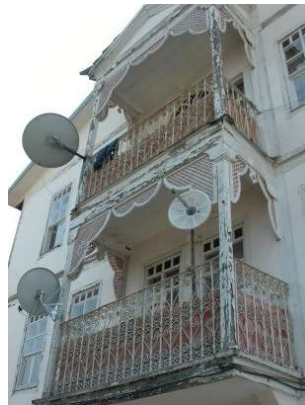
Figure 3.78. Pre-intervention views of Çakırlar house, east facade (Çetin,Y, 2006, p.550)
