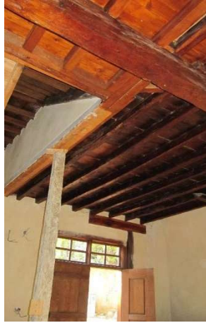
Figure 4.59. Current view of the GPOI03 that indicate the G.R1 (Author, 2013)
