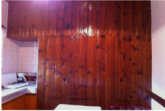
Figure 3.96. Post-intervention view of FPOI03 at second floor (Author, 2013)
