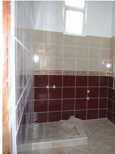
Figure 3.95. Post-intervention view of FPOI02 (taken from the Taraklı Municipality, 2013)
