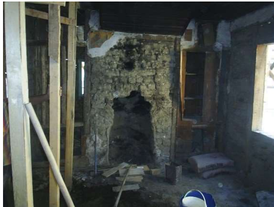
Figure 4.38. G.R1 is a removal of original fireplace in GPOI08 (taken from the Taraklı Municipality, 2013)
