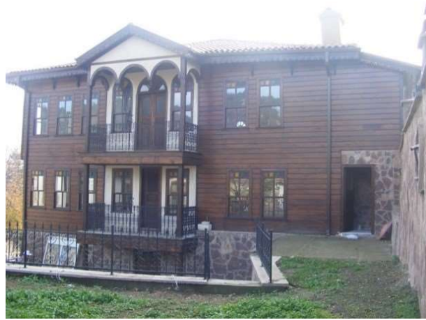
Figure 4.26. Post-intervention view of north side facade (Author, 2013)
