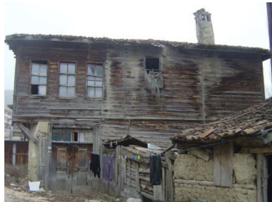
Figure 3.55. Pre-intervention view of Hacı Rıfatlar house, west facade (Özkan, 2008, p.125)
