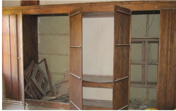
Figure 4.67. Alterations of closets at second floor of the house (Author, 2013)
