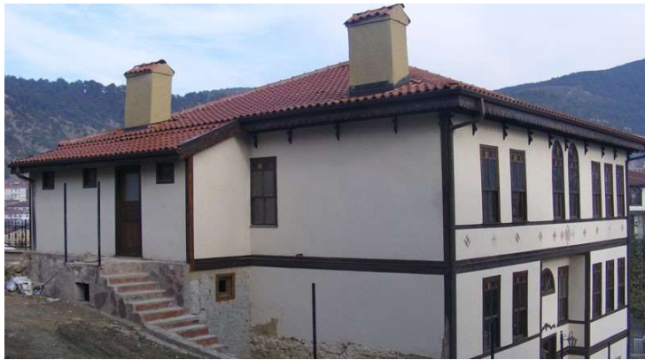
Figure 4.29. Post-intervention view of west facade (Author, 2013)
