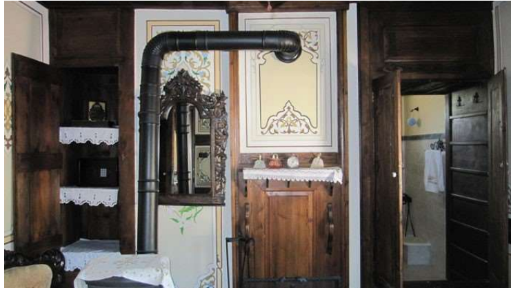
Figure 3.24. Closet, fireplace and gusülhanes' current condition (Author, 2013)
