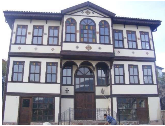
Figure 3.11. Post-intervention view of Kadirler house, east facade (Author, 2013)
