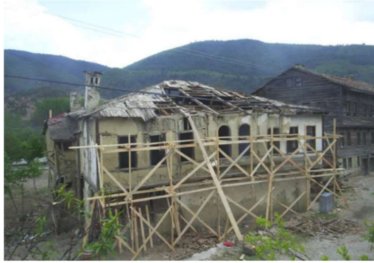
Figure 3.53. Pre-intervention view of Hacı Rıfatlar house, north facade (Özkan, 2008, p.187)
