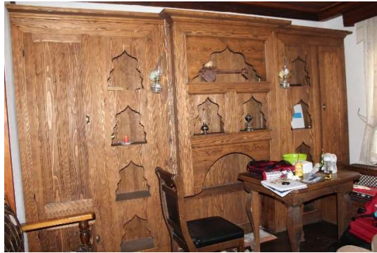
Figure 4.37. G.A2, Alteration of closet during the hotel transformation (Author, 2013)
