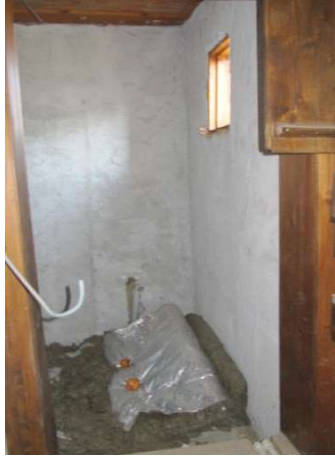
Figure 4.64. Alteration of wet spaces in first floor (Author, 2013)
