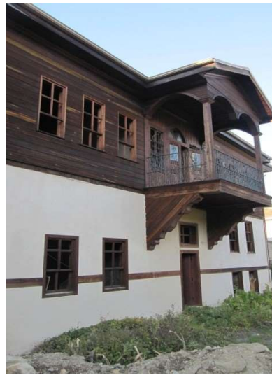
Figure 3.60. Post-intervention view of Hacı Rıfatlar house, south facade (Author, 2013)
