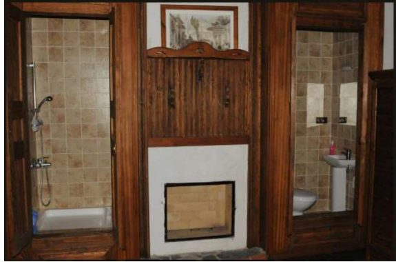
Figure 4.46. F.A1, alteration of fireplace and closets in room FPOI09 (taken from the Taraklı Municipality, 2013)
