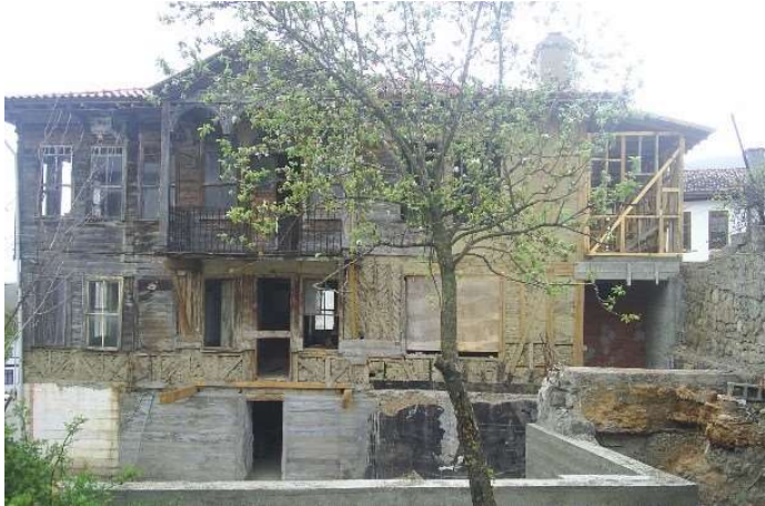
Figure 4.27. Pre-intervention view of north side facade (taken from the Taraklı Municipality, 2013)
