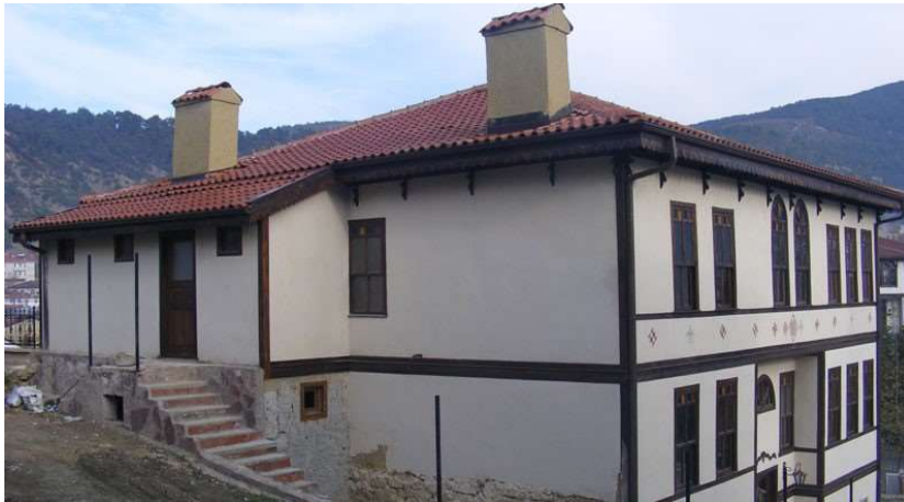
Figure 4.21. S.AD1, Mass addition of wet space and AD2. Addition of outdoor staircase to the existing building (Author, 2013)
