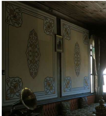
Figure 4.10. A.2, post-intervention view of kalemîşi works on the walls of ground floor (Author, 2013)
