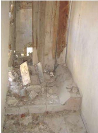
Figure 4.65. Pre-intervention view of wet spaces in first floor (Özkan, 2008)
