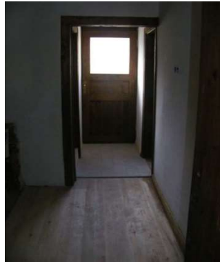
Figure 4.18. S.A2, Alteration of a wall. The new door was opened on the indicated wall (taken from the Taraklı Municipality, 2013)
