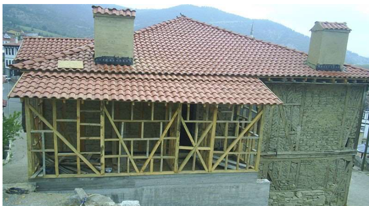
Figure 4.30. Pre-intervention view of west facade (Author, 2013)
