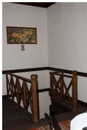
Figure 3.48. Post-intervention view of staircase, FPOI08 (Author, 2016)
