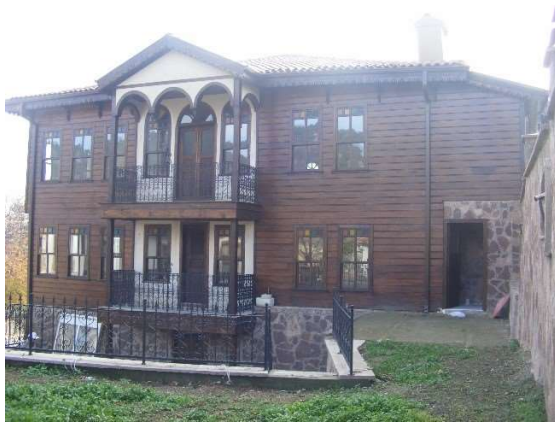
Figure 3.14. Post-intervention view of Kadirler house, north facade (Author, 2013)
