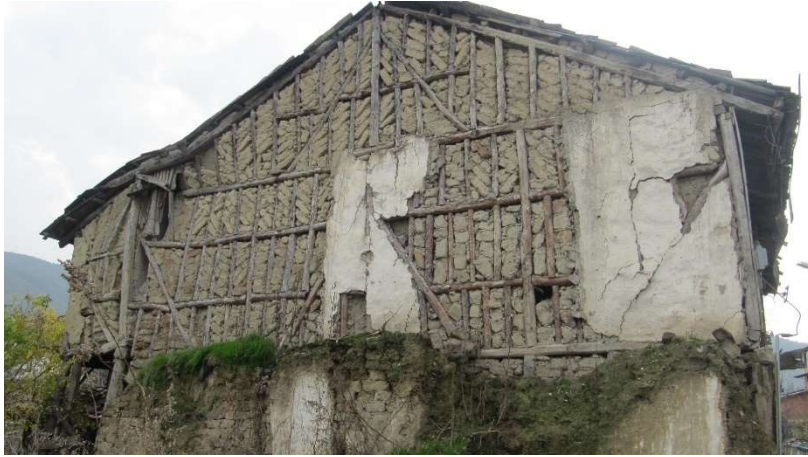
Figure 2.14. Timber skeleton system with mudbrick infill from unnamed house in Taraklı (Author, 2016)
