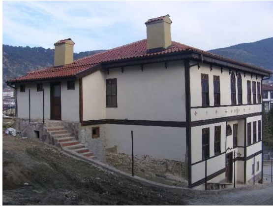
Figure 3.13. Post-intervention view of Kadirler house, west facade (Author, 2013)
