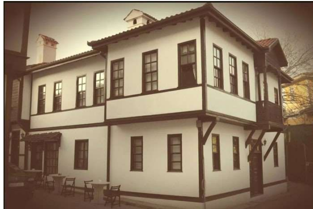
Figure 3.34. West facade of Abdi İbrahim house (taken from the Taraklı Municipality, 2016)
