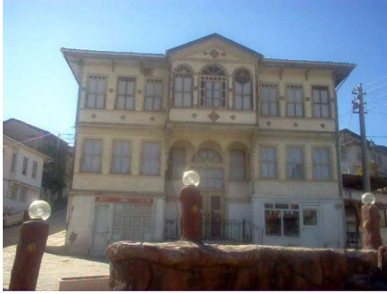
Figure 4.24. Pre-intervention view of west side facade (taken from Taraklı Municipality archives, 2013)
