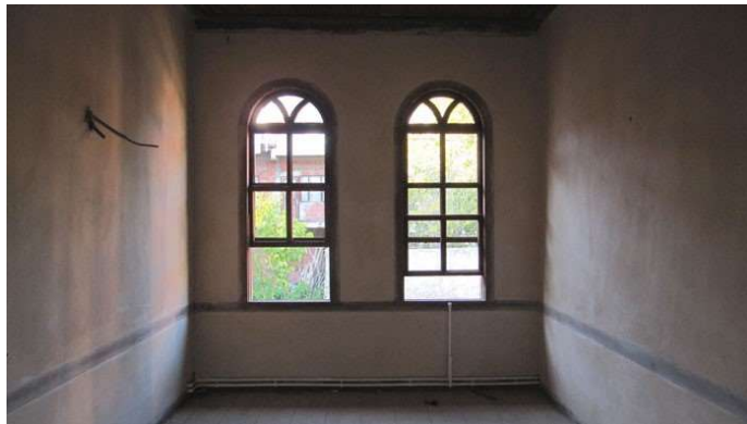
Figure 3.73. Post intervention of eyvan on second floor after its transformation (Author, 2013)
