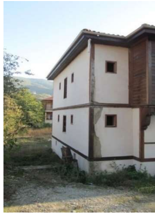
Figure 3.62. Post-intervention view of Hac1 Rıfatlar house, east facade (Author, 2013)
