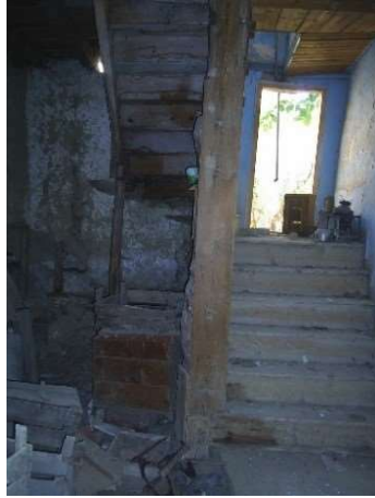
Figure 4.43. Pre-intervention views of GPOI02 (taken from the Taraklı Municipality, 2013)
