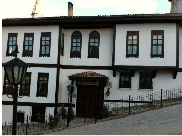
Figure 3.82. Post-intervention view of Çakırlar house, north facade (Author, 2013)
