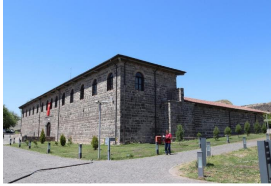
Figure 46. The Prison building from the southeast side, 2019.
