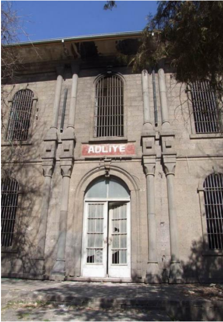
Figure 57. The entrance of Courthouse, before restoration.
