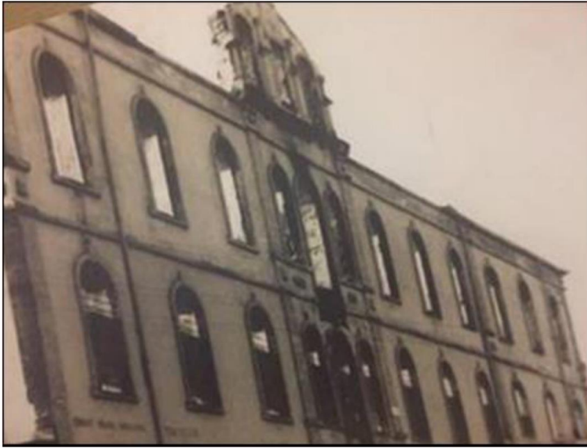
Figure 35. The damaged condition of Industrial School, n.d.
