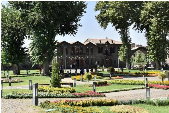
Figure 71. The north facade of Defterdarlık ve Vakıflar buildings, 2019.
