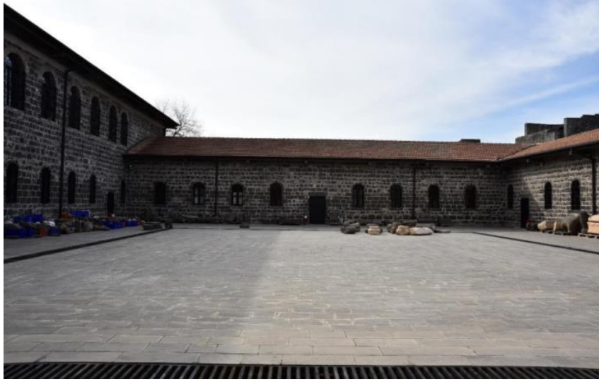
Figure 45. The view from the courtyard of Prison building, 2019. (İş, 2019, p. 274.)
