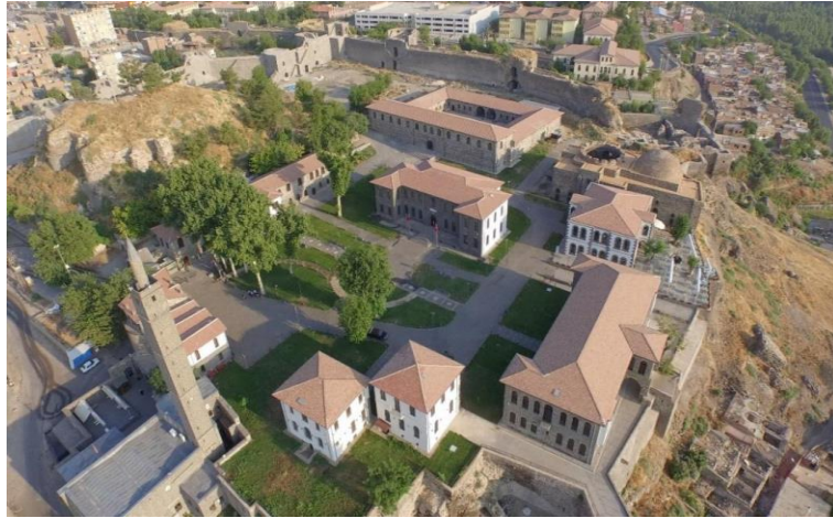
Figure 39. The current state of the administrative center in the citadel.
