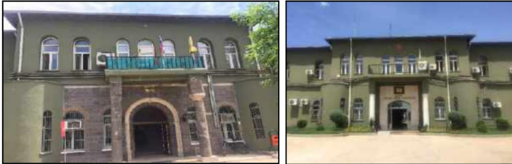
Figure 30. The west and east entrance facades of the barracks building, n.d. (Payaslı Oğuz and Halifeoğlu, 2019, p. 485)
