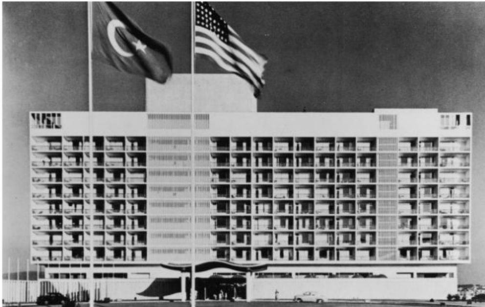
Fig. 10. Istanbul Hilton Hotel (1952–55), designed by the US architectural firm Skidmore, Owings & Merrill with Sedad Hakkı Eldem as the local collaborating architect
